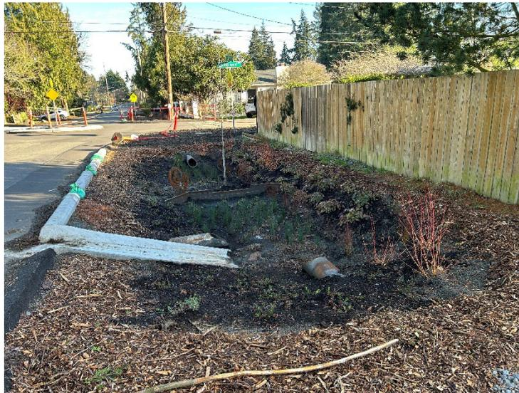
**Figure 4-12. Looking East from 24th Ave SW and SW Kenyon St – The New Bioretention Facility, Walkway, and Bridge**
