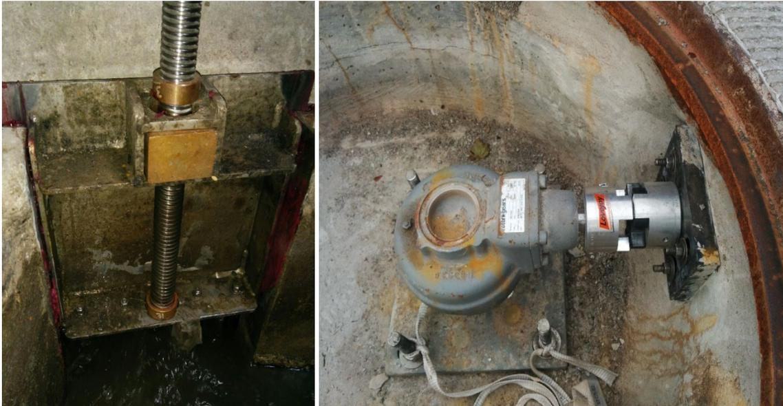
**Figure 4-1. New Basin 99 Sluzice Gate (Left) and Actuator Motor (Right)**
