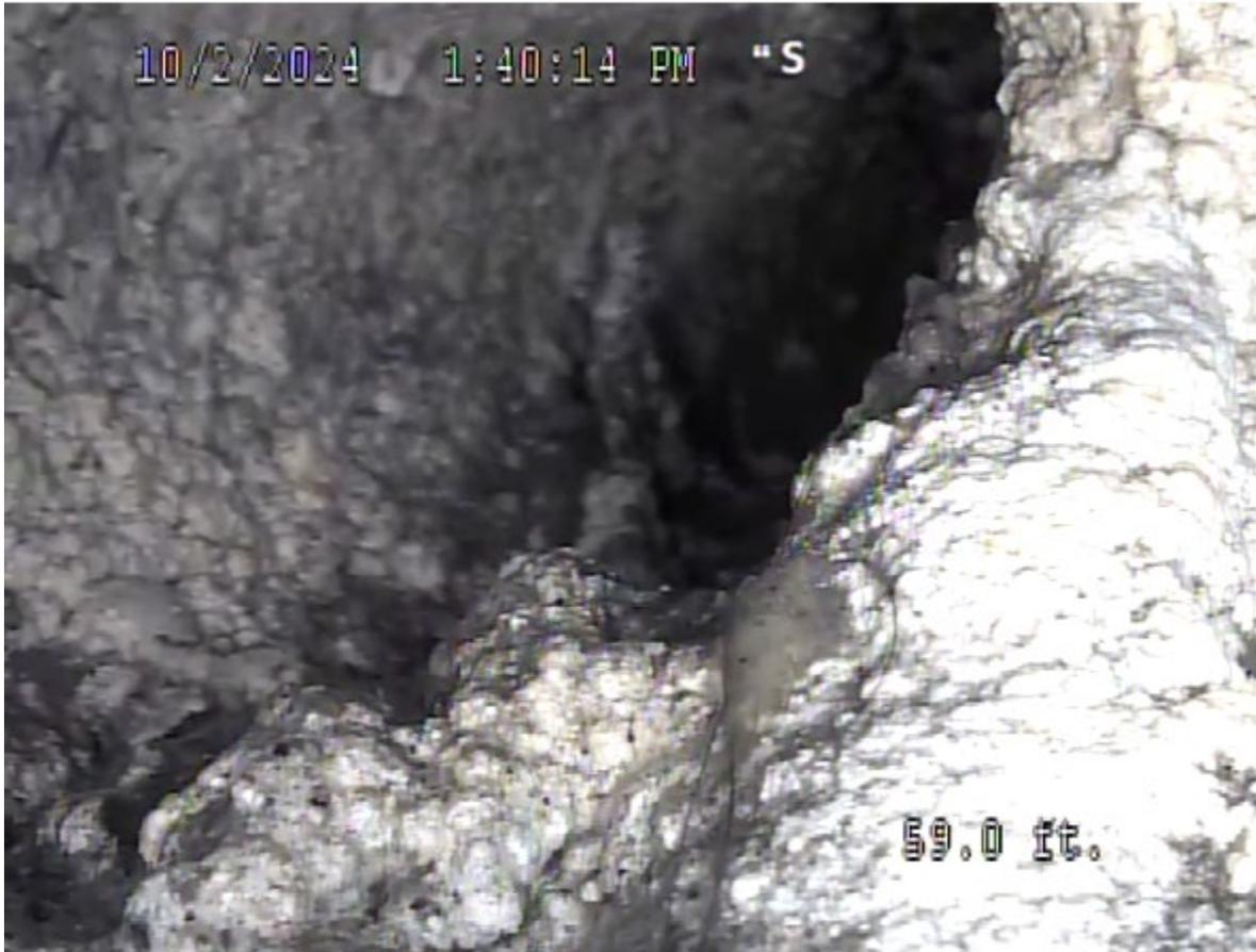
Figure 3-1. 2024 Mainline Image Demonstrating Visible FOG Accumulations Resulting in SSO Near the University of Washington
