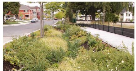
Figure 2. A completed natural drainage system
