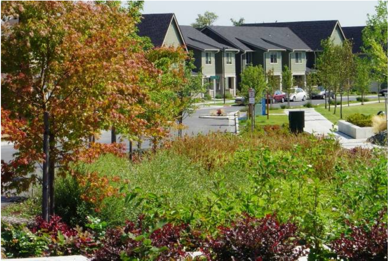
Drainage swales cleanse rainwater runoff and contribute to the site's beauty
