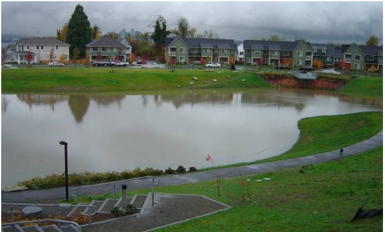
The stormwater pond is surrounded by art elements and a walking trail.
