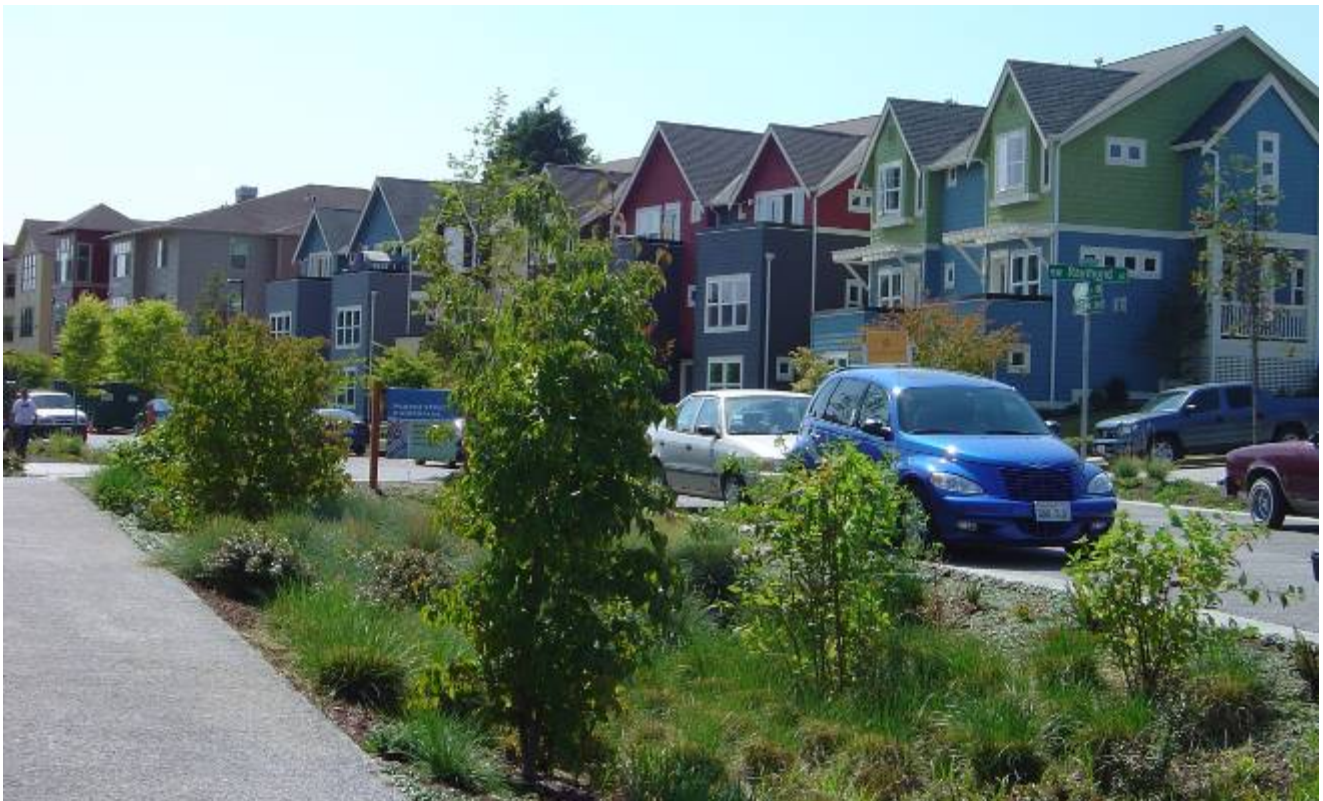
Porous pavement sidewalk and street, drainage swale, homeowner units
