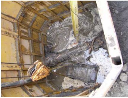
Figure 3-4 Boiling Sands Along the Duwamish
