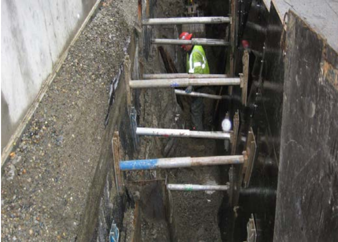
Figure 3-12 Excavation Next to a Building
