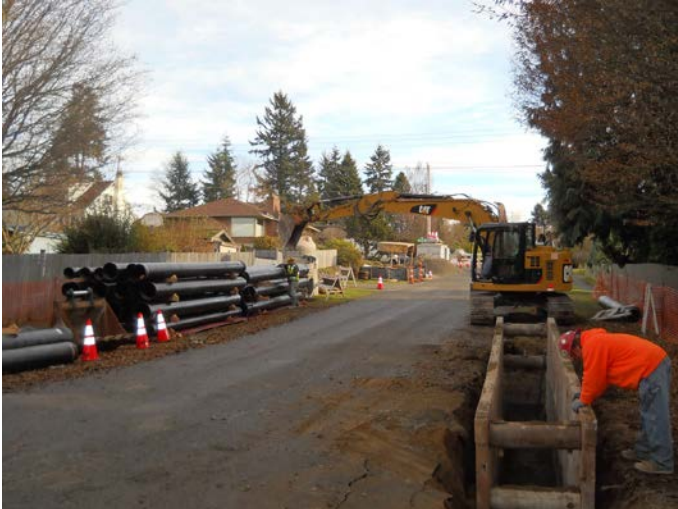
Figure 3-7 Trench Box Without Ground Support
