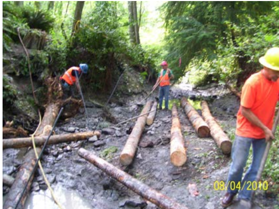
Figure 3-15 Hand-carried Logs for Stream Structure
