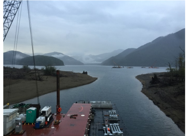
Figure 3-18 In-Water Barge Operations on Chester Morse
