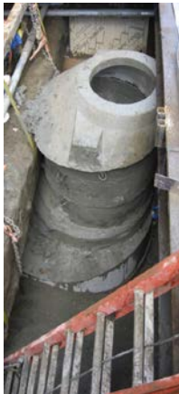
Figure 3-5 Offset MH Cone Between 2 Ducts
