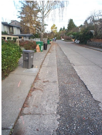
Figure 3-21 Temporary Crushed Rock Pavement
