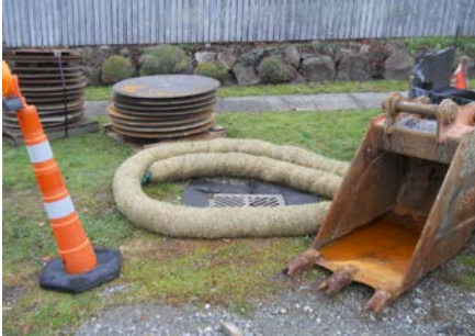
Figure 3-2 Compost Sock Around Grate Outside of Travel Lane
