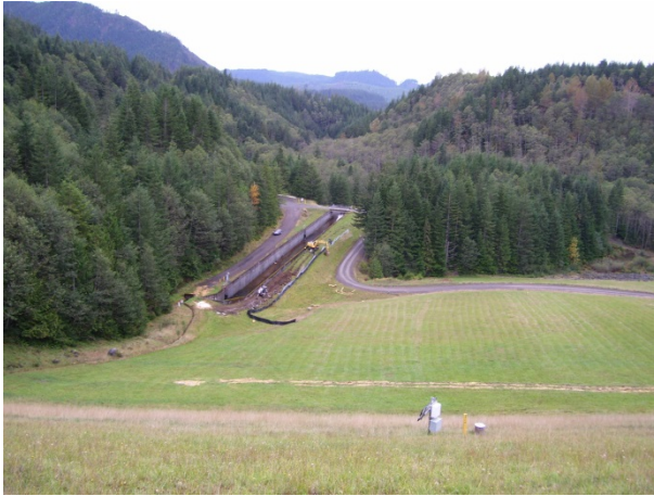
Figure 3-17 Conduit Installation on Tolt Dam Lake
