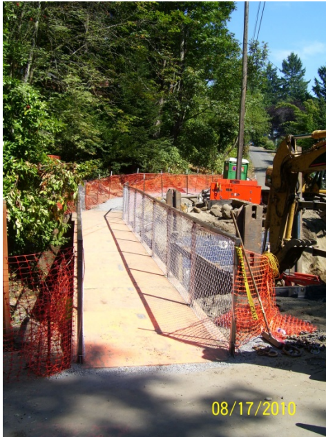
Figure 3-20 Temporary Pedestrian Bridge
