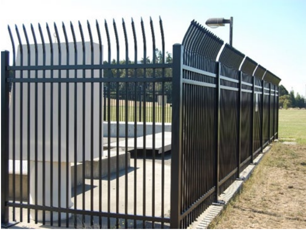
Figure 15-6 Estate Ornamental Fencing
