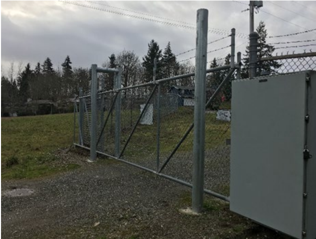
Figure 15-11 Anti-Ram Protected Gate
