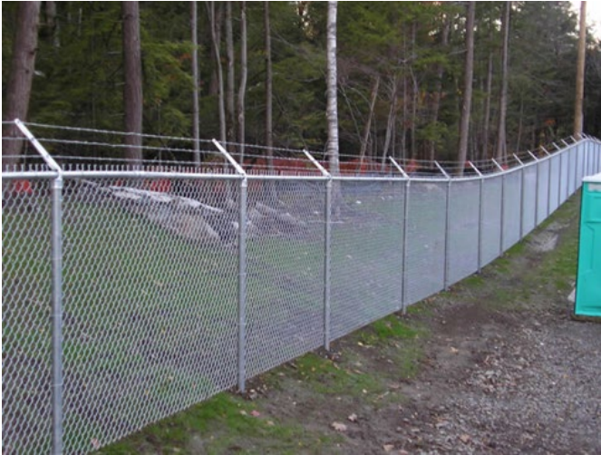
Figure 15-5 Chain-Link Fencing
