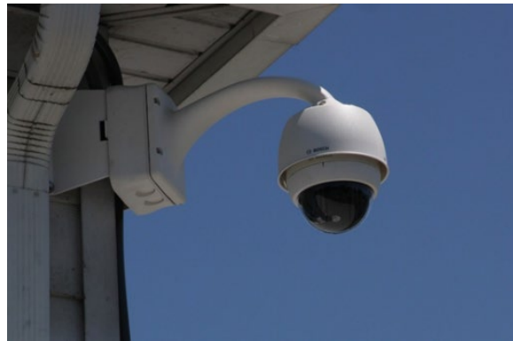
Figure 15-14 PTZ/Dome Camera
