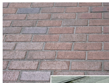
New brick is compatible with existing brick.
