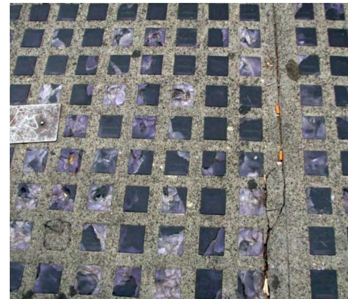
Existing areaway glass blocks on Maynard Ave. S.
