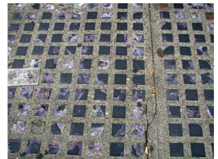
Existing glass areaway blocks
