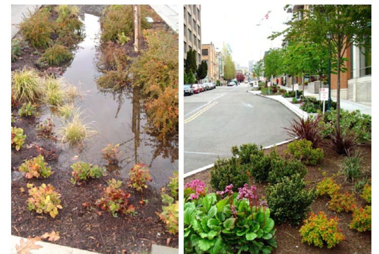
Stormwater raingarden and abundantly planted curb bulb
