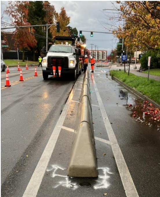
Toronto-style barrier being installed in Seattle
