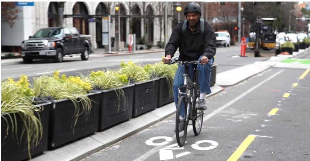
Two-way protected bike lane with planters
