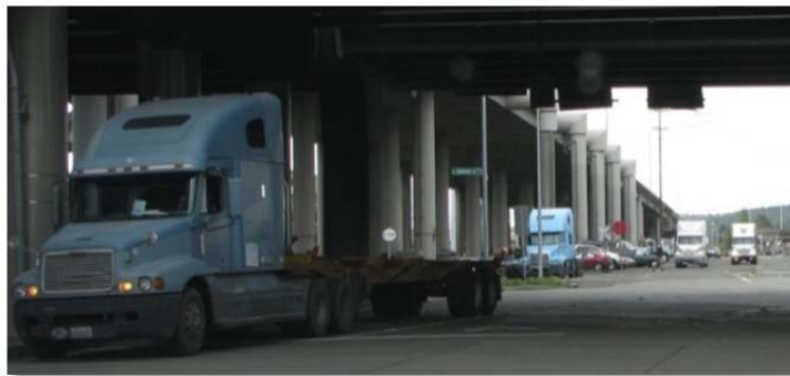
East Marginal Way provides major truck connections to support freight mobility and goods movement
