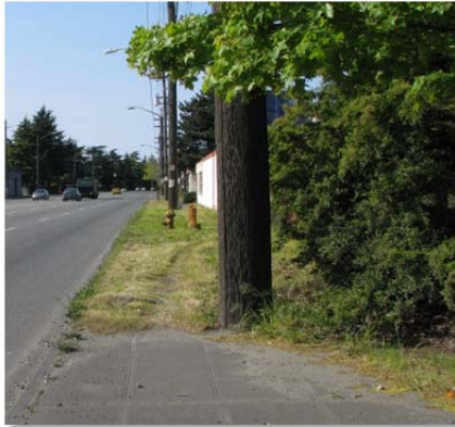
Incomplete sidewalk network along the south portion of the corridor
