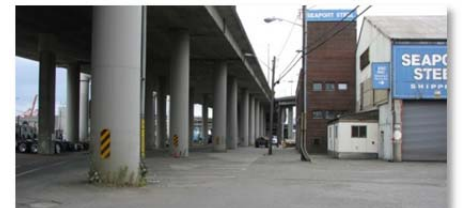
There are no delineated pedestrian paths along the Center Transition Segment
