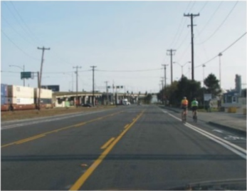
North segment has sidewalk on west side and bike lanes on both sides with buffer of varying width.
