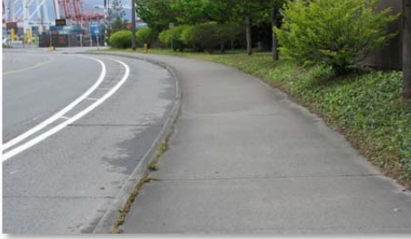
Varying buffer between the bike lanes, sidewalk, and vehicle lanes along the North Segment
