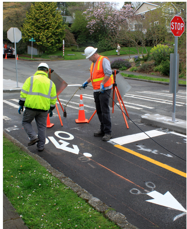
Workers installing a cycle track (protected bicycle lane).
