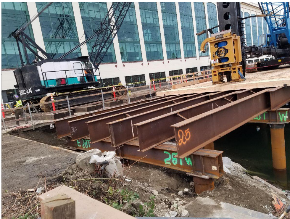
Construction of temporary trestle for Fairview Bridge
