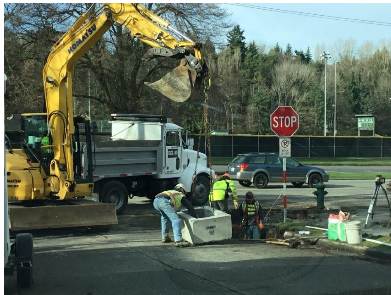
Construction on Green Lake Way N
