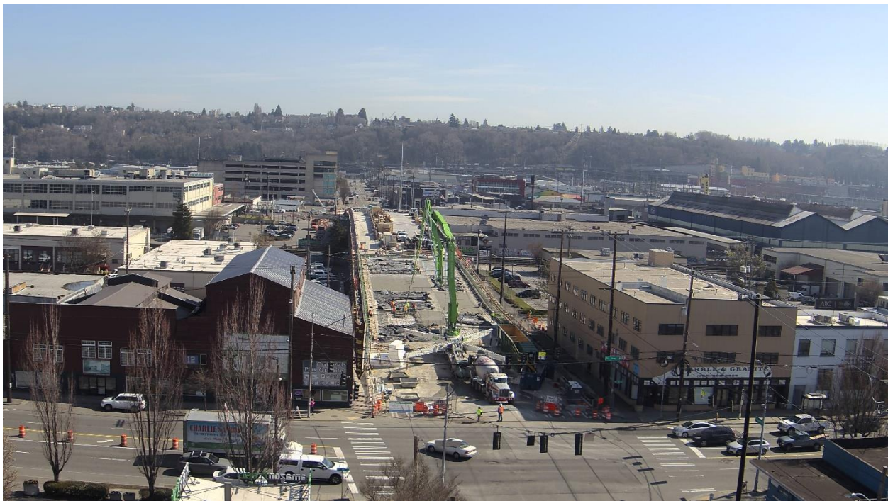
The Lander Overpass continues to take shape
