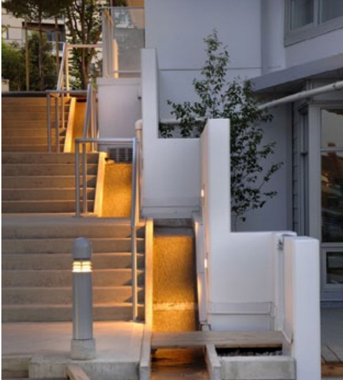
Integrated lighting for an outdoor stair (Photo: Vince Klassen; Design: Perkins+Will)
