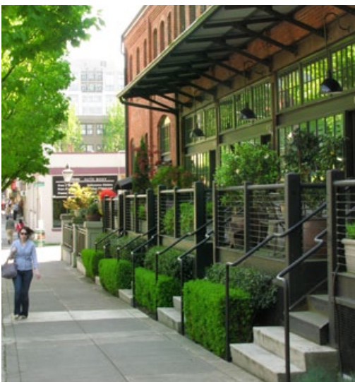
Exemplary compact residential frontage This narrow threshold makes a good transition from the public to private realm in a small amount of space. The railings and deck plants strike a balance between the desire to screen and the need for visual connection to the sidewalk. (Photo: Don Vehige)
