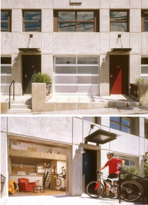
Vertical separation and direct access Two views of the same frontage. Garage doors allow a connection between private interior and patio space, adjacent to the shared space of a pedestrian pathway. Well articulated entrances, stairs, and patios mediate the sloping site and the transition from public to private. Landscaped walls between units articulate individual units and provide a sense of privacy to each patio. (Photo: Steve Keating Photography; Design: GGLO)
