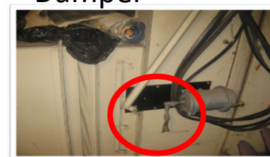
Disconnected Damper
