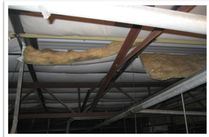
Failed roof insulation
