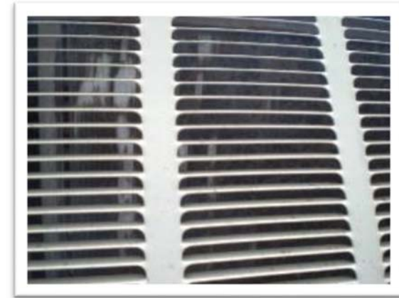
Clean any coils that are dirty to increase efficiency of the unit
