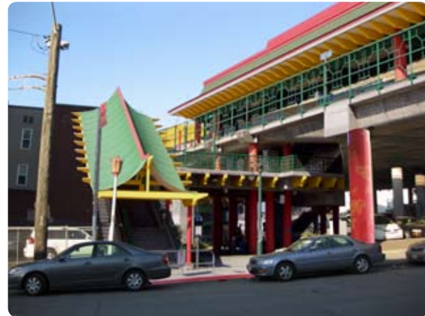
The space below I-5 as light rail station
