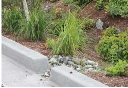
Densely landscaped with native plants, this swale is designed to hold street run-off and release it slowly into the stormwater system.
