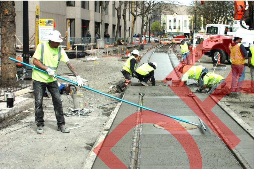
Raked tine concrete finish
