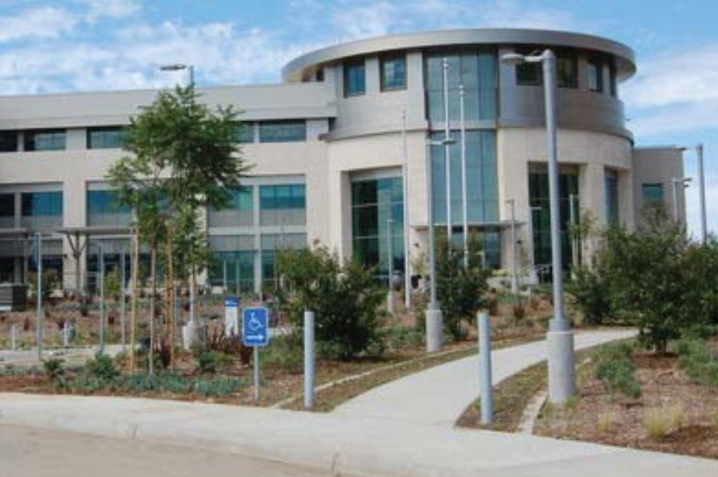
El Cajon Public Safety Building
