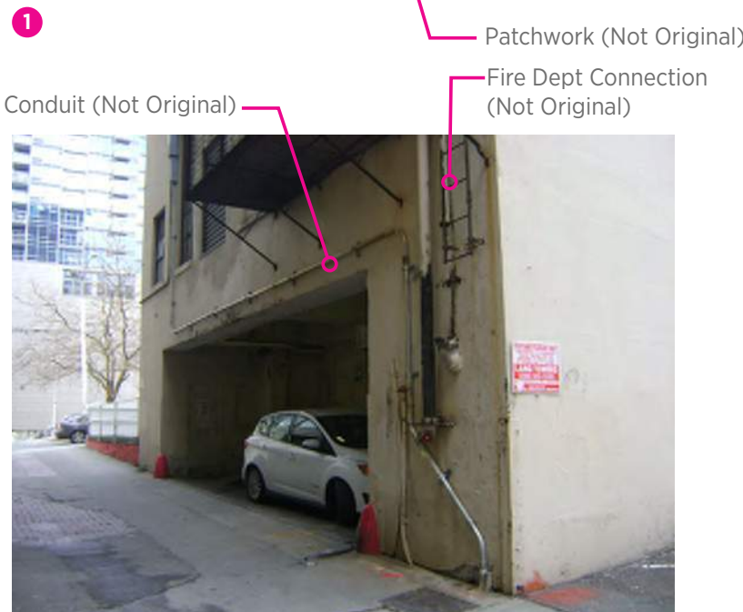
2 Damaged Facade Materials and Mech. System Upgrades
