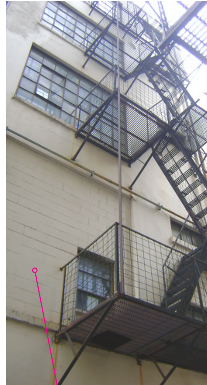
3 CMU Infill (Not Original)
