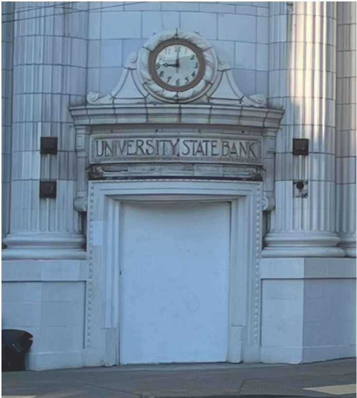
1. PRESENT CONDITIONS: THE SOUTHWEST VESTIBULE IS CURRENTLY FRAMED CLOSED WITH PAINTED PLYWOOD AND IS INACCESSIBLE.
