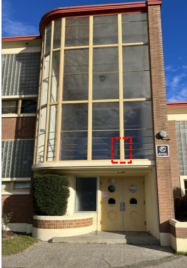
Fixed windows at stairwells
