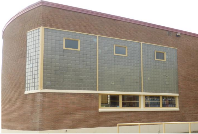
Fixed windows in glass block walls
