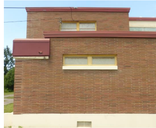
Narrow fixed windows
