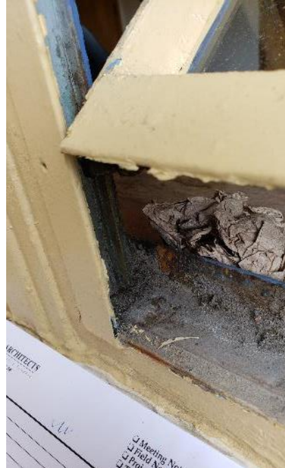
Photo above depicts an exterior view at the corner of in-swing hopper.
