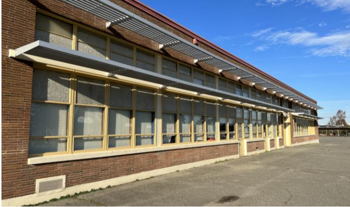
Shop windows and doors
