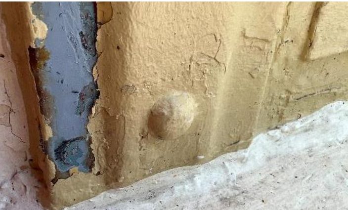
Epoxy repair at corroded corner
