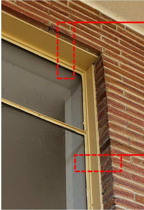
Head flange against steel ledger angle
