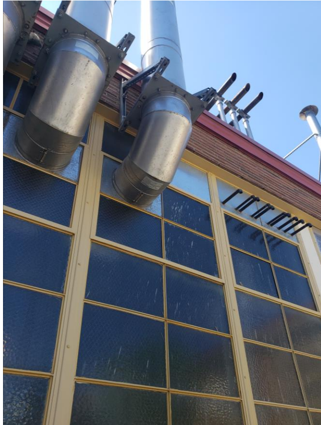
Infill of glazing for ductwork and pipe penetrations
