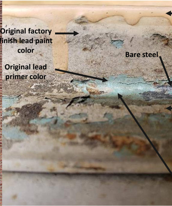
Close-up photo above depicts the various current and historic paint finishes.
