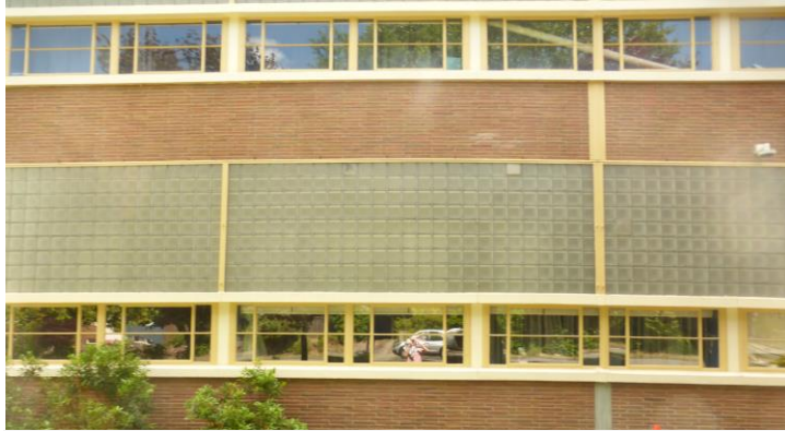
Classroom windows with combination in-swing hopper and fixed sides
