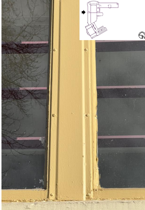
Wider steel mullions at stairwells
