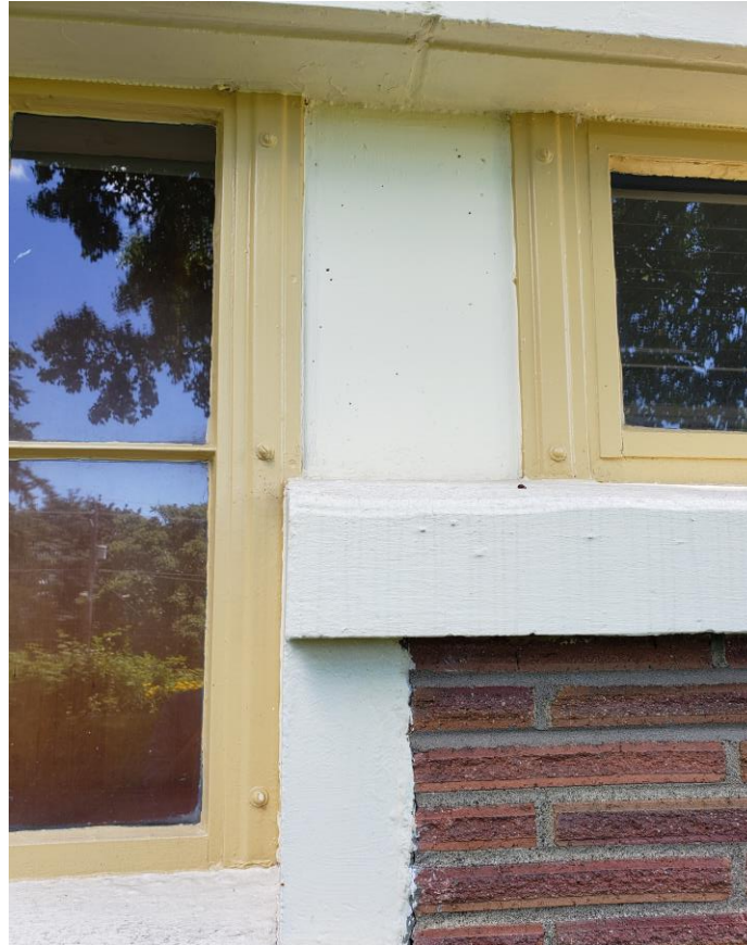
Notched steel mullion around transition in concrete ledge
