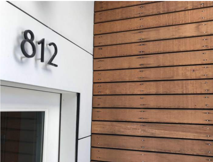
Fiber Cement Panel & Cedar Rainscreen Transition
