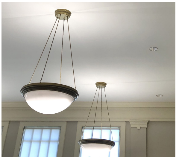
Relamp existing pendant fixtures and replace existing recessed downlights, typical throughout upper level
