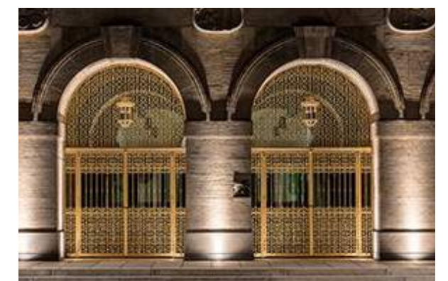
Dimmable in-grade uplights to give landmark building a nighttime presence
