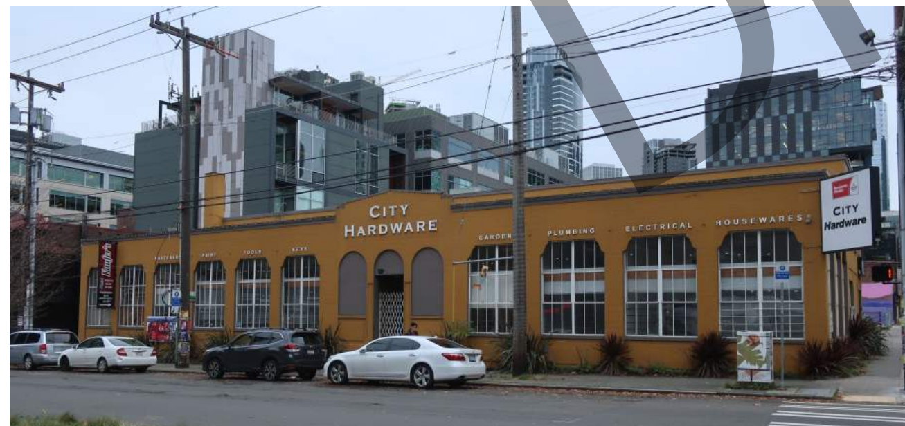
North facade, along Harrison Street
