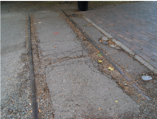
6. tracks create uneven pavement at the entry
