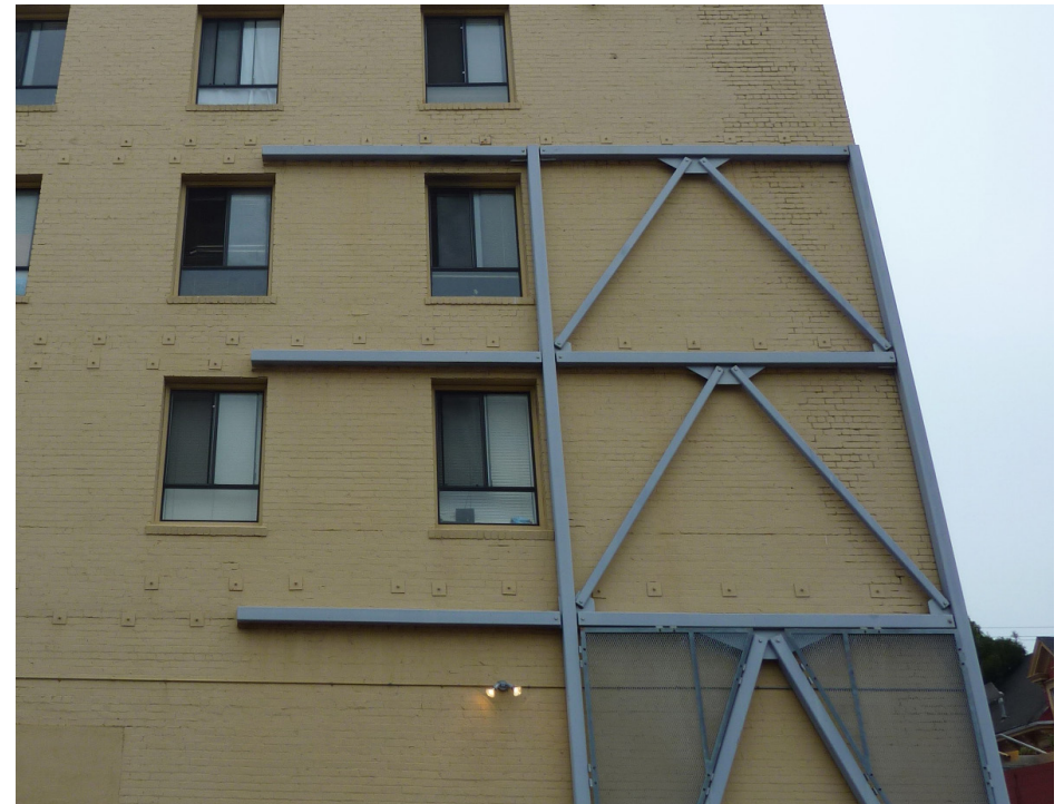
Example of seismic retrofit of masonry wall
