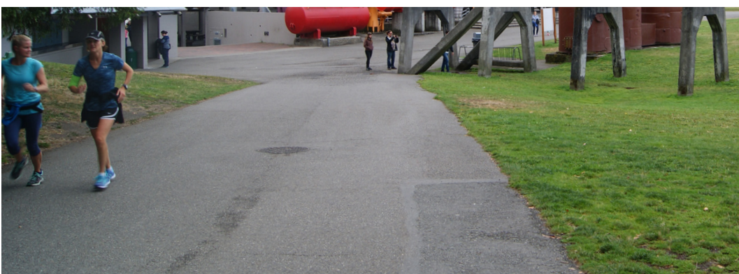
4. walkway is inaccessible due to cross slope
