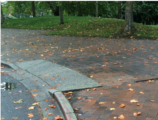
3. curb ramp slope is inaccessible
