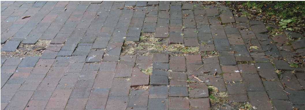
7. inaccessible routes due to uneven paving
