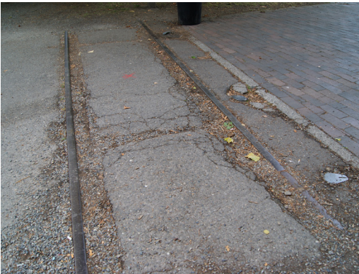
6. tracks create uneven pavement at the entry
