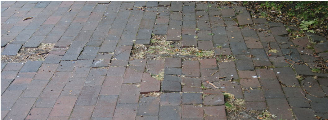
7. inaccessible routes due to uneven paving
