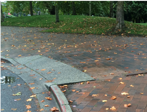
3. curb ramp slope is inaccessible
