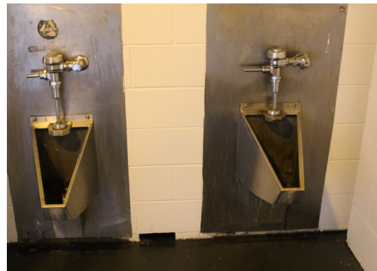
8. inaccessible urinal due to no elongated rim
