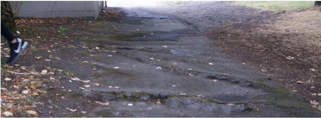
5. tree roots create uneven pavement at ADA pathway
