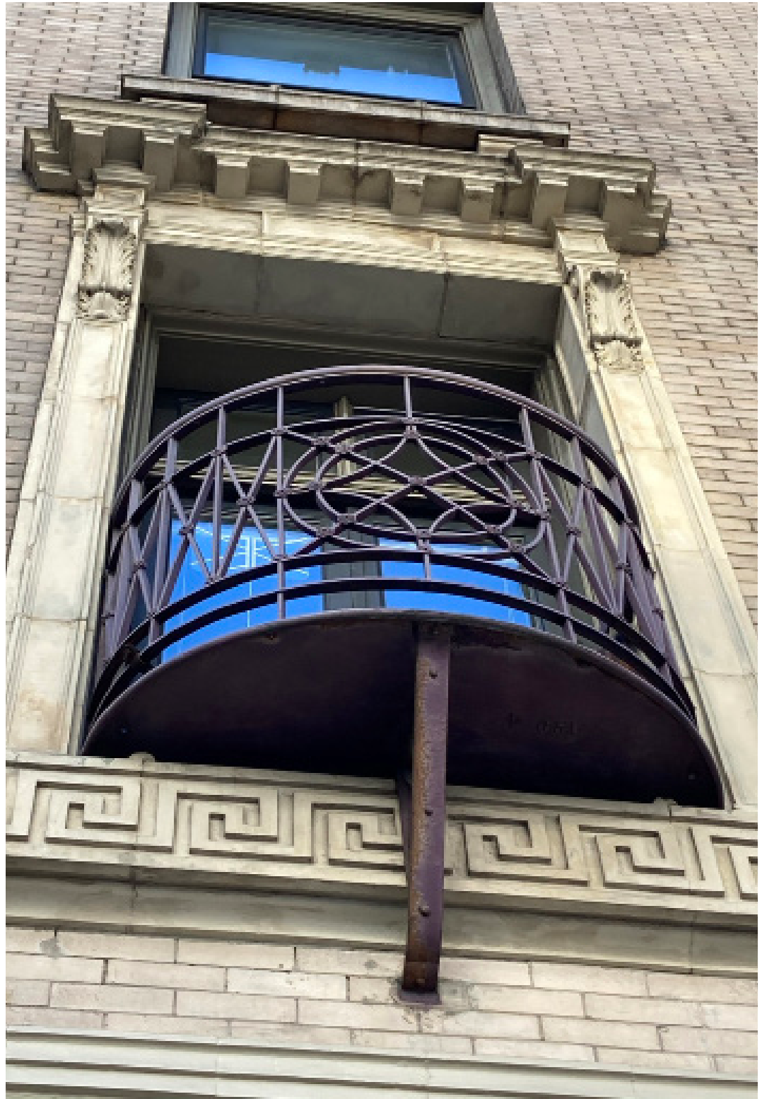
Juliet Balcony - East Facade
