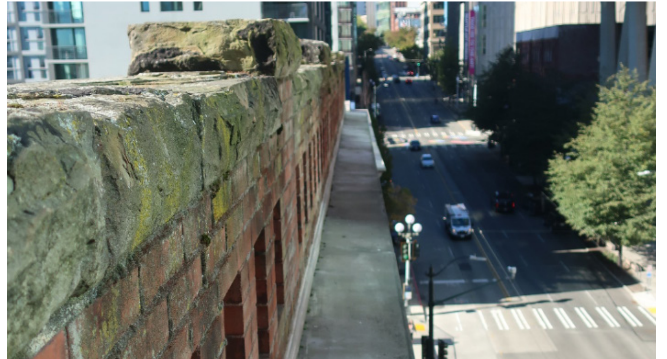
Parapet Wall - Exterior View Facing North
