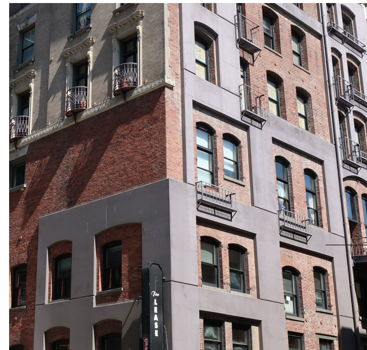
Concrete Shear Wall
