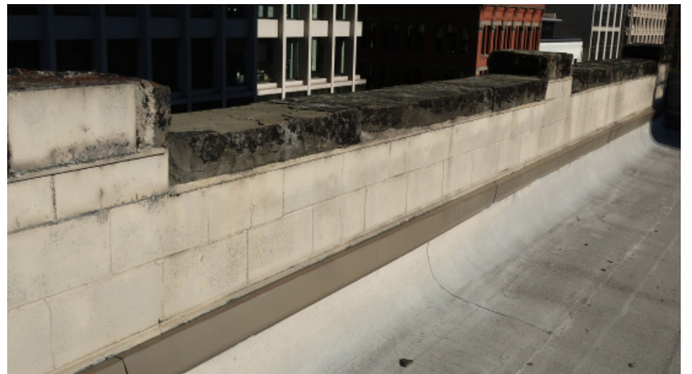
Parapet Wall - Roof View Facing Southeast
