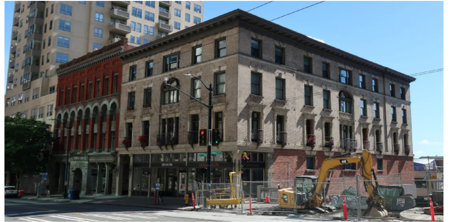
East and North Facades
