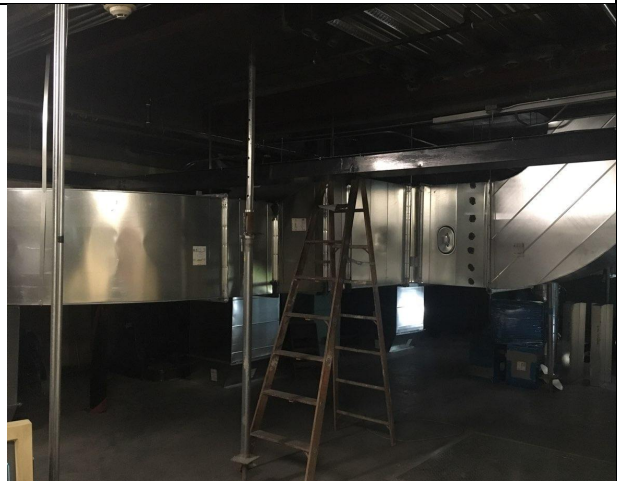
Ductwork for Elevator Pressurization
