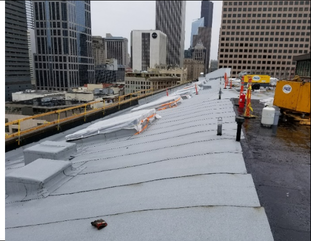
New Roof w/ Insulation Under
