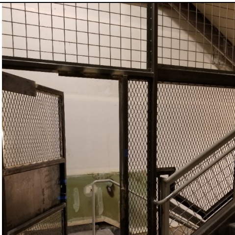
Stair Separation Gates
