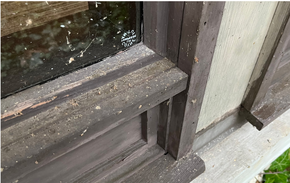
1. STOREFRONT GLAZING SYSTEM: WOOD FRAMED WITH FIXED SINGLE PANE GLASS, WINDOW GROUPING TYPICAL THROUGHOUT. 2.DETAIL OF SOUTH FACING WOOD STOREFRONT FRAME WITH SINGLE GLASS PANE
