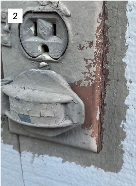
1&2. THE SIDING IS 3/4"X 5 1/2" TONGUE AND GROOVE CEDAR. BUILDINGS HAVE BEEN PAINTED MULTIPLE TIMES SOME AREAS HAVE BEEN PAINTED ONCE, OTHER AREAS UP TO THREE TIMES. THE FIRST PAINT COLOR WAS MEDIUM GRAY/BEIGE. THE CURRENT COLOR FOR MOST OF THE BUILDINGS IS A DARK GREEN/GRAY COLOR 3. UNDERSIDE OF ROOF EAVE IS 3/4"X 5 1/2" TONGUE AND GROOVE CEDAR STAINED DARK BROWN.
