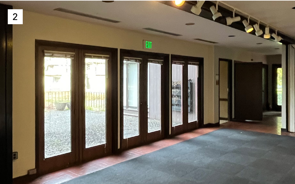
1&2. DOORS ARE WOOD WITH SINGLE PANE FULL LITES AND DARK HARDWARE THAT MATCHES THE COLOR OF THE WINDOW FRAMES. DOOR FRAMES ARE WOOD PAINTED DARK BROWN TO MATCH RAILINGS AND WOOD WINDOW FRAMES.
