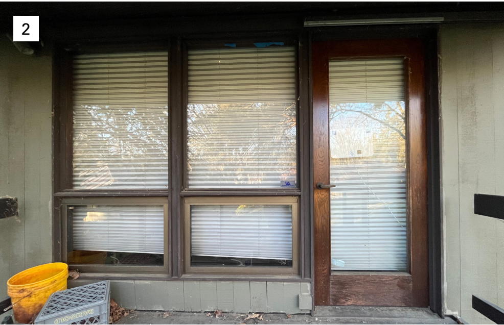
1. EXISTING WINDOWS ARE DOUBLE PANE GLASS IN WOOD FRAMES PAINTED DARK BROWNTO MATCH RAILINGS AND DOOR FRAMES. 2.THE OPERABLE CASEMENT WINDOWS AND AWNING WINDOWS ARE ALUMINUM FRAMED INSET IN PAINTED WOOD FRAMING.
