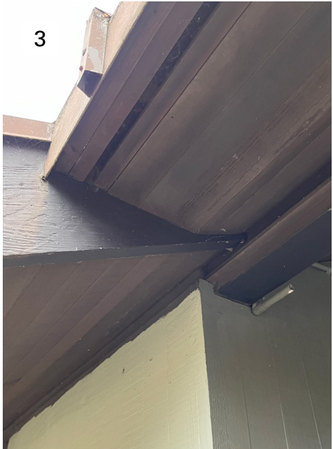
1&2. THE SIDING IS 3/4"X 5 1/2" TONGUE AND GROOVE CEDAR. BUILDINGS HAVE BEEN PAINTED MULTIPLE TIMES SOME AREAS HAVE BEEN PAINTED ONCE, OTHER AREAS UP TO THREE TIMES. THE FIRST PAINT COLOR WAS MEDIUM GRAY/BEIGE. THE CURRENT COLOR FOR MOST OF THE BUILDINGS IS A DARK GREEN/GRAY COLOR 3. UNDERSIDE OF ROOF EAVE IS 3/4"X 5 1/2" TONGUE AND GROOVE CEDAR STAINED DARK BROWN.
