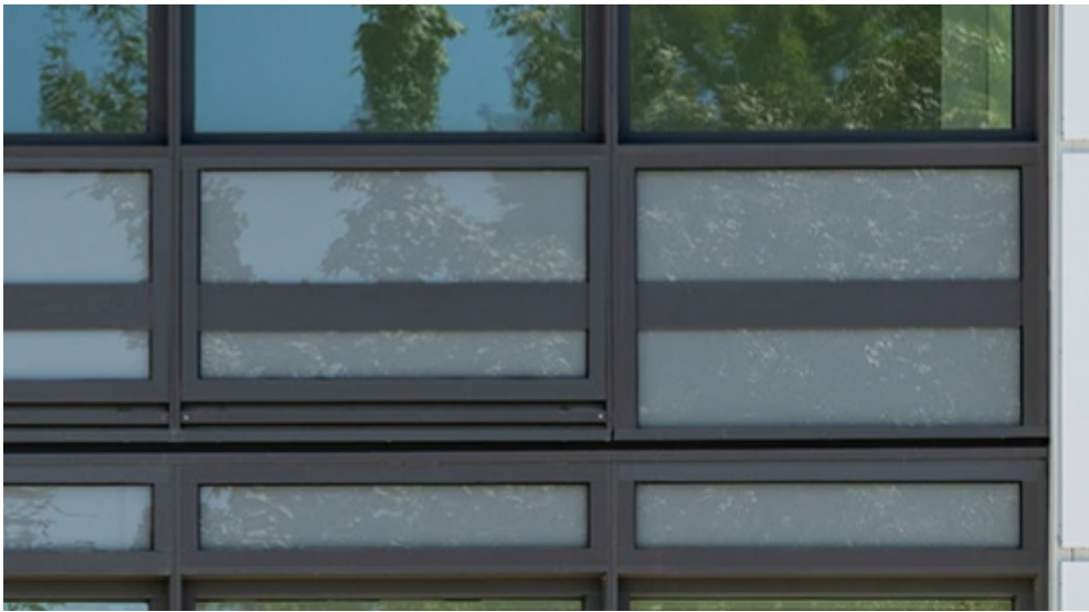
CASCADIA UNIVERSAL SERIES THERMALLY BROKEN FIBERGLASS STOREFRONT FRAMES AND WINDOW UNITS WITH COLORS AND PROFILES SIMILAR TO EXISTING WINDOW UNITS
