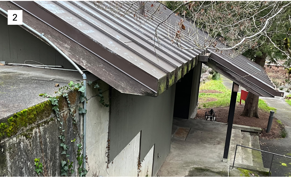
1. BATTEN SEAM METAL ROOFS ARE FINISHED WITH A DARK BROWN PAINT.THE PAINT IS PEELING IN MANY LOCATIONS.
