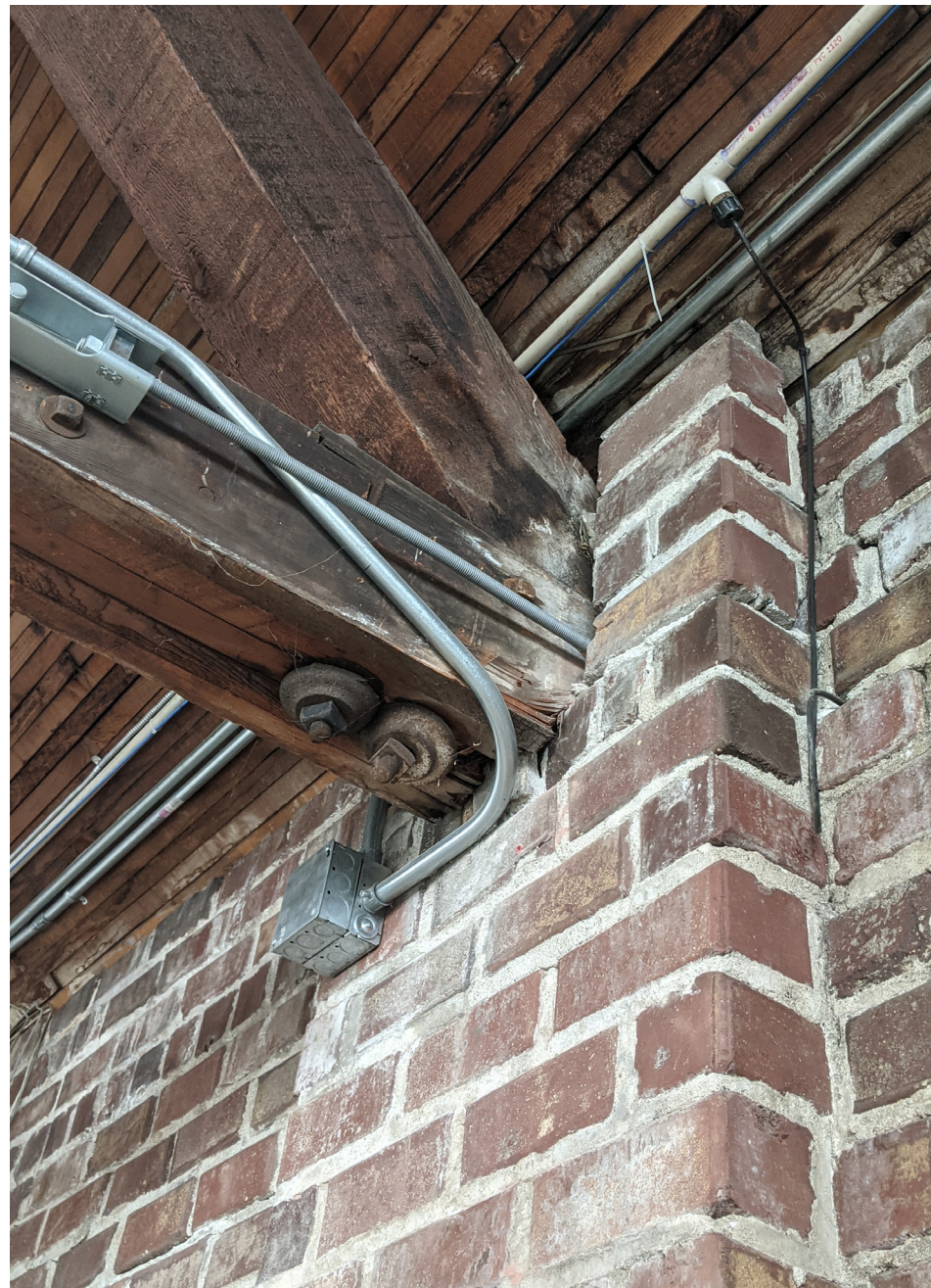
Existing interior conditions - truss, NLT roof and brick
