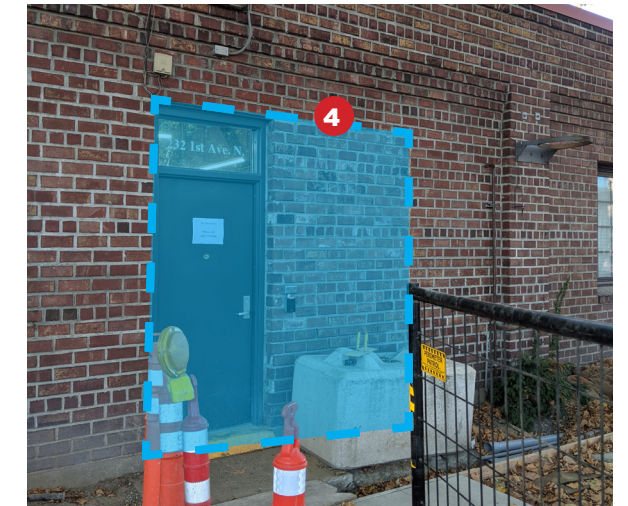
North facade - existing conditions
