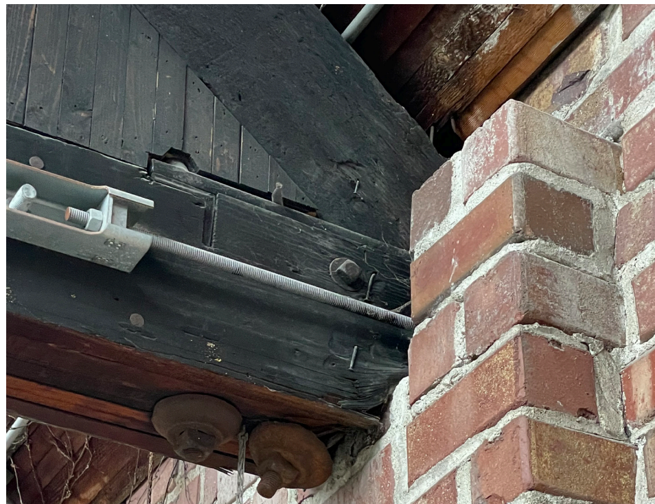
Existing truss condition at courtyard
