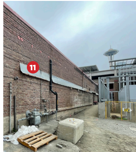
South Facade - existing conditions
