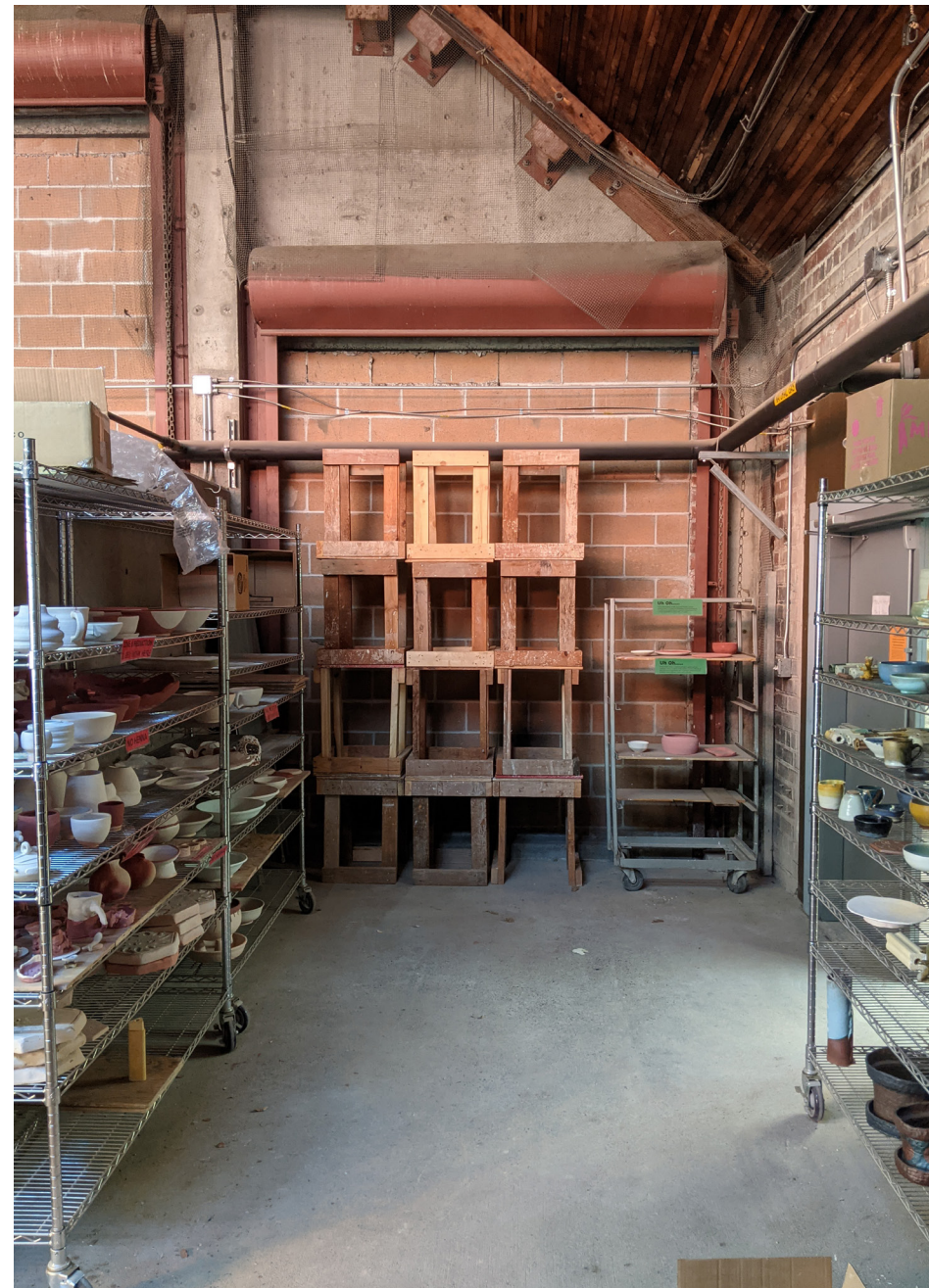
Existing interior conditions - former Pottery NW space looking E
