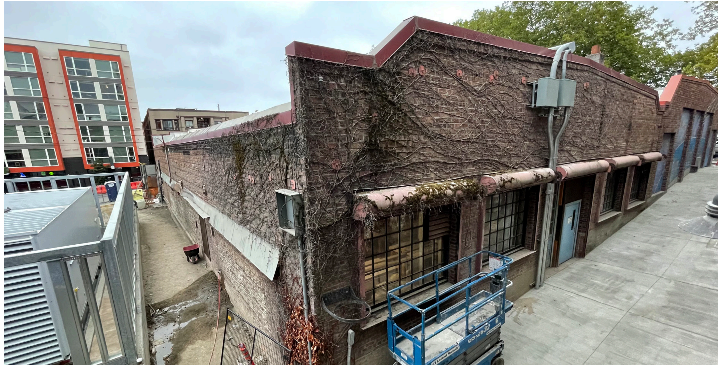
Southeast corner along existing alley
