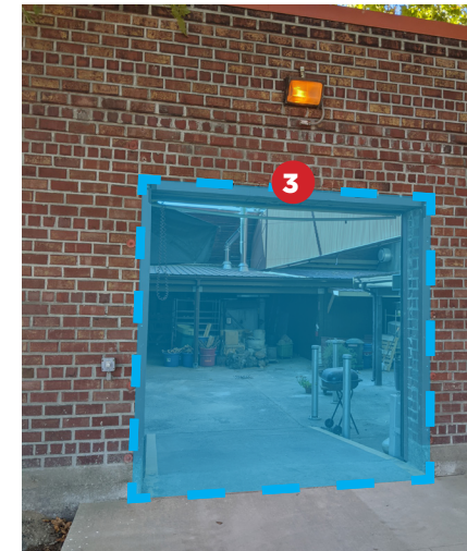
North facade - existing conditions
