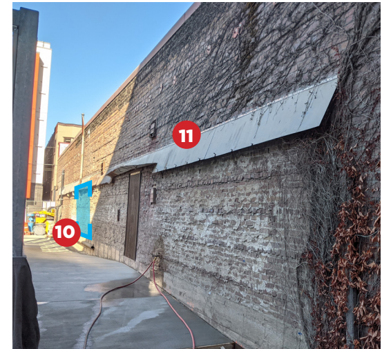
South Facade - existing conditions
