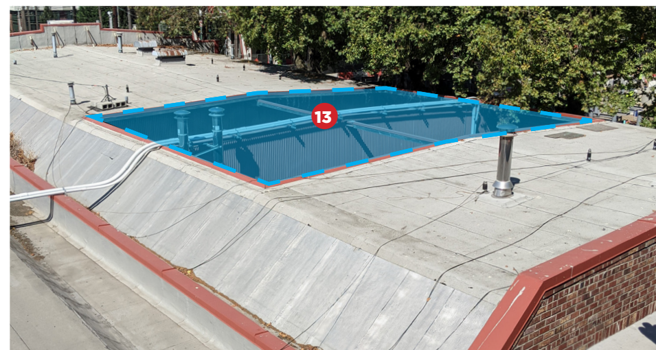
Roof - existing conditions
