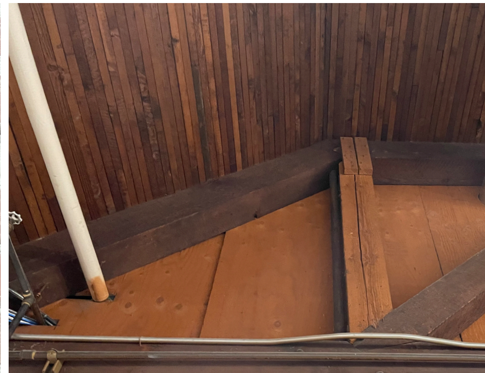
Historic truss and roof deck
