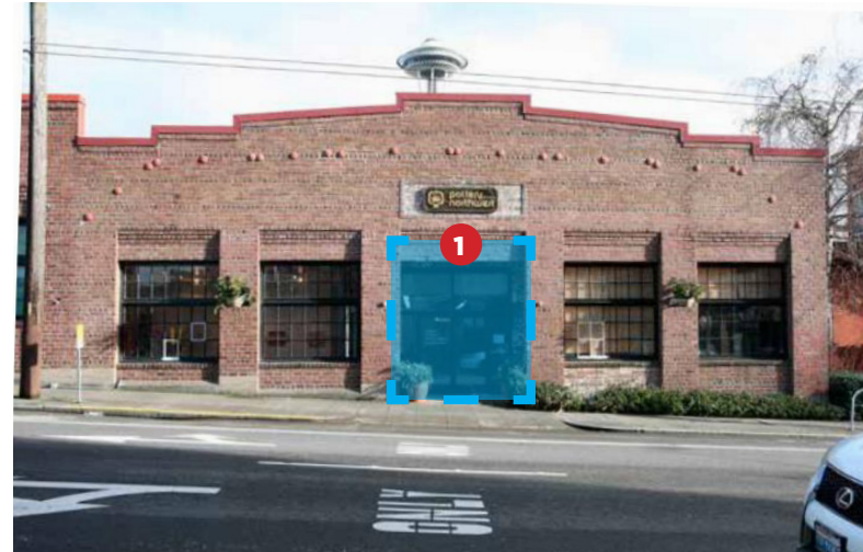
South building - existing conditions
