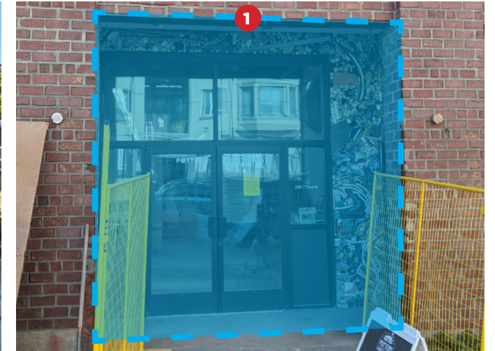
South building - existing conditions
