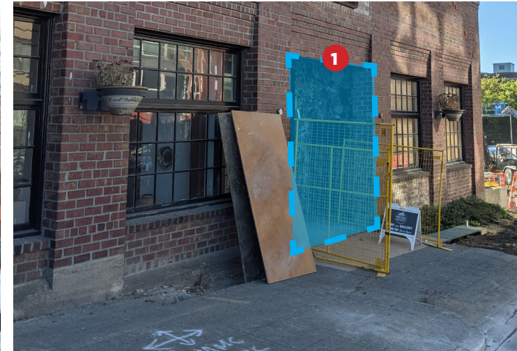
South building - existing conditions
