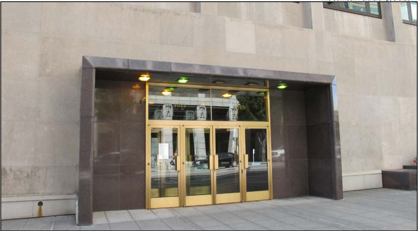
Figure 14 • Federal Reserve Bank, Seattle, eastern façade detail
