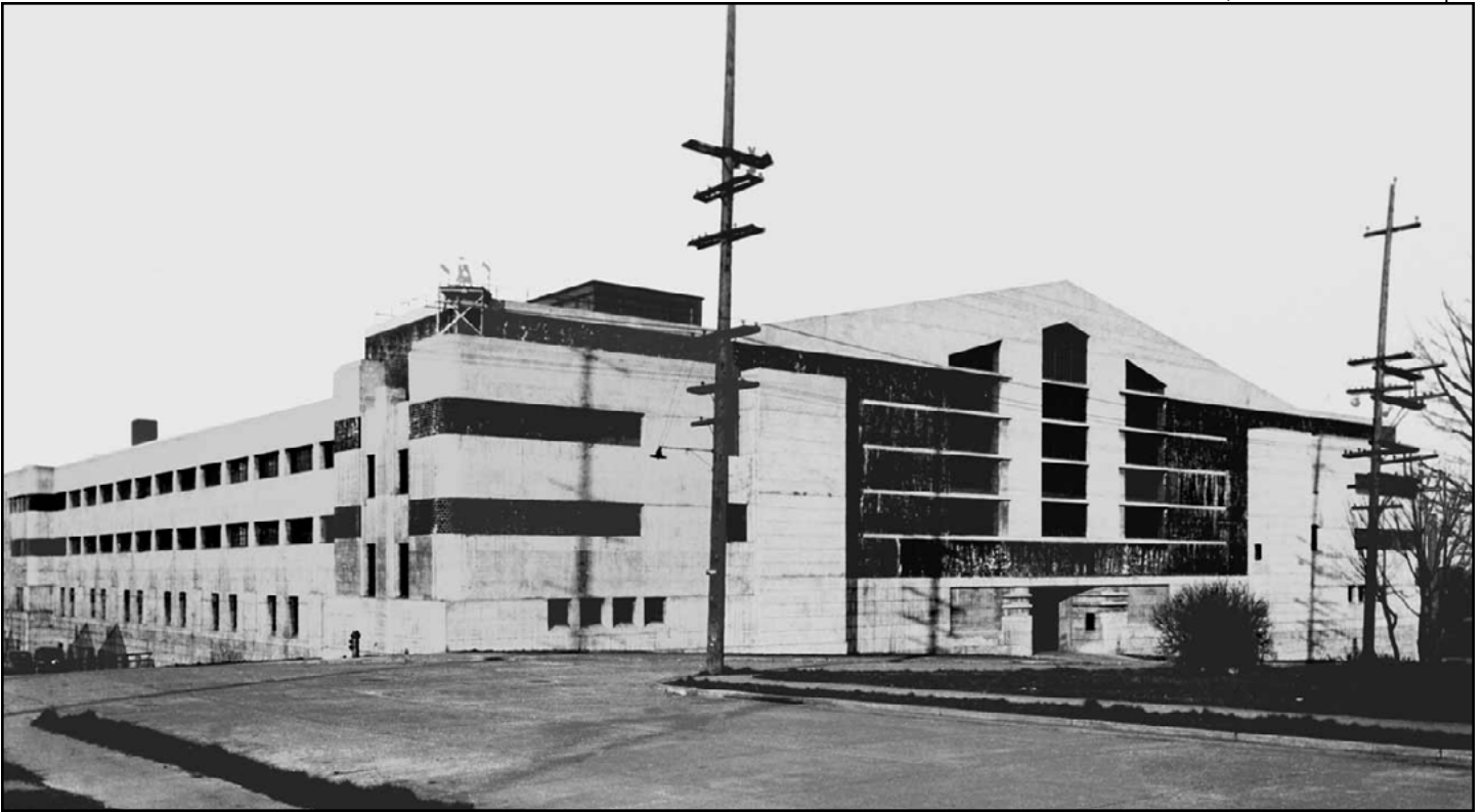
Figure 37 • Washington National Guard Armory (1939, Naramore and Young, altered)
