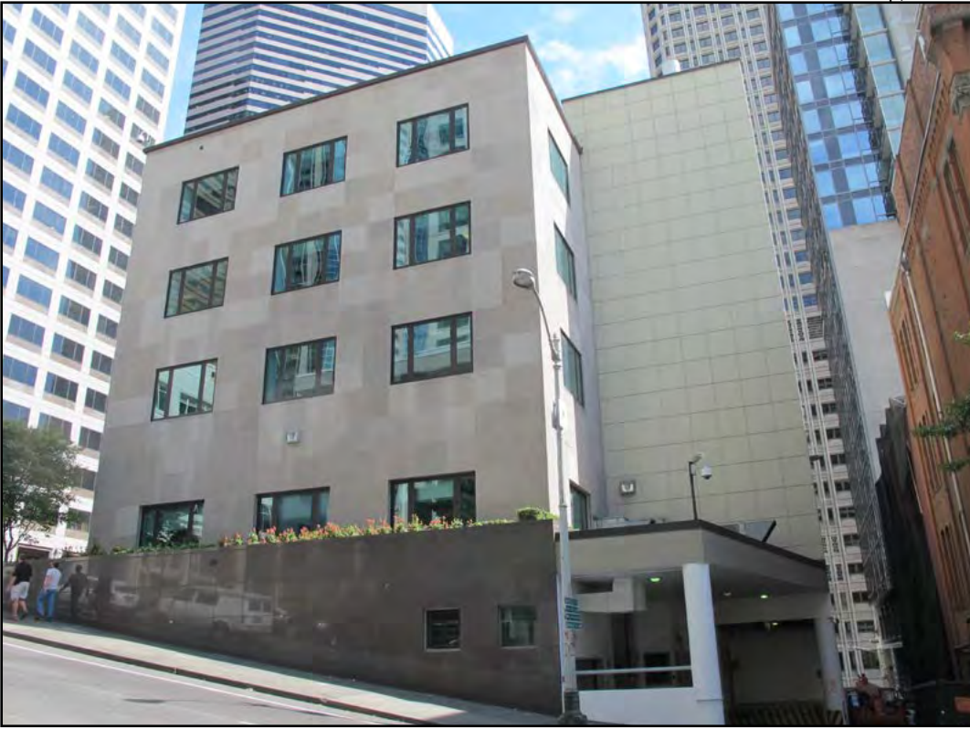
Figure 17 • Federal Reserve Bank, Seattle, northern façade
