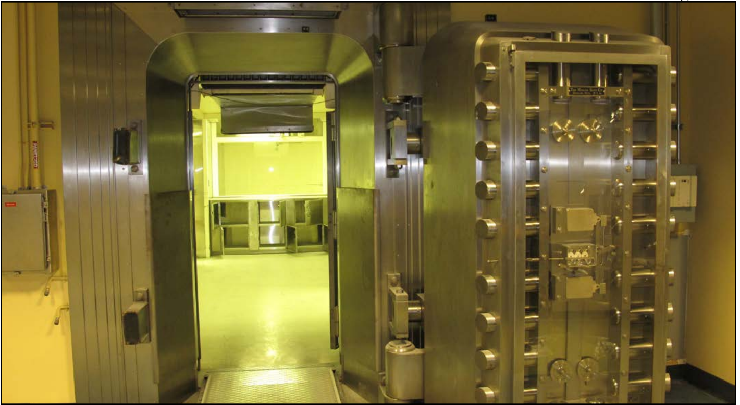
Figure 21 • Federal Reserve Bank, Seattle, vault at ground floor
