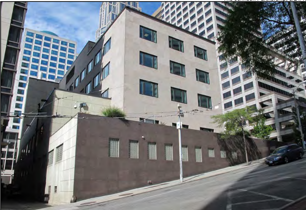
Figure 16 • Federal Reserve Bank, Seattle, southern façade
