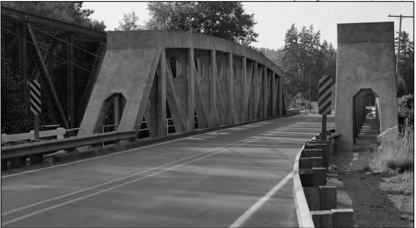
Figure 42 • McMillin Bridge spanning the Puyallup River (1934, George Runciman, engineer)
