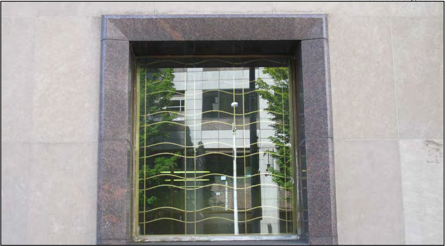
Figure 13 • Federal Reserve Bank, Seattle, eastern façade detail
