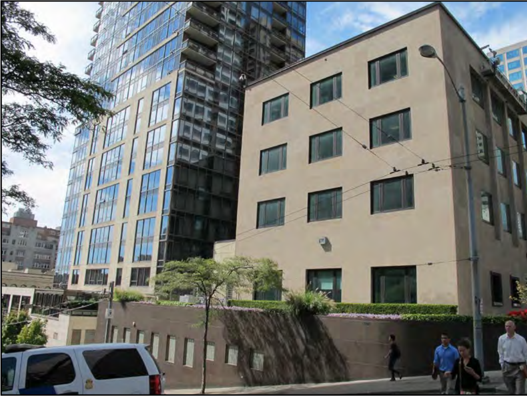
Figure 15 • Federal Reserve Bank, Seattle, southern façade
