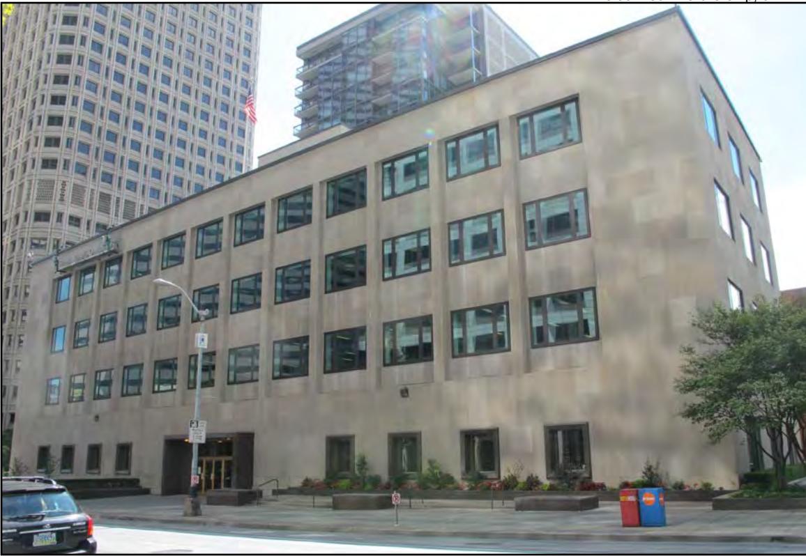
Figure 11 • Federal Reserve Bank, Seattle, eastern façade
