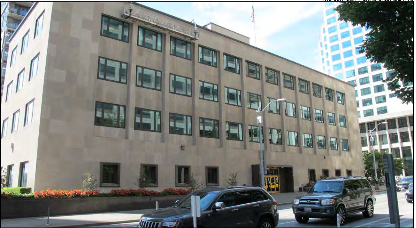
Figure 12 • Federal Reserve Bank, Seattle, eastern façade
