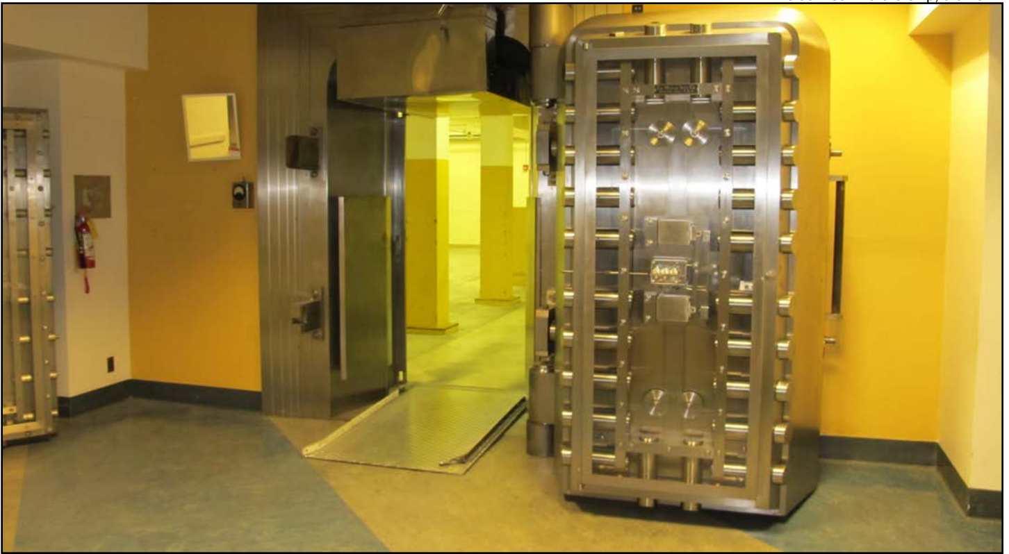
Figure 19 • Federal Reserve Bank, Seattle, vault at basement
