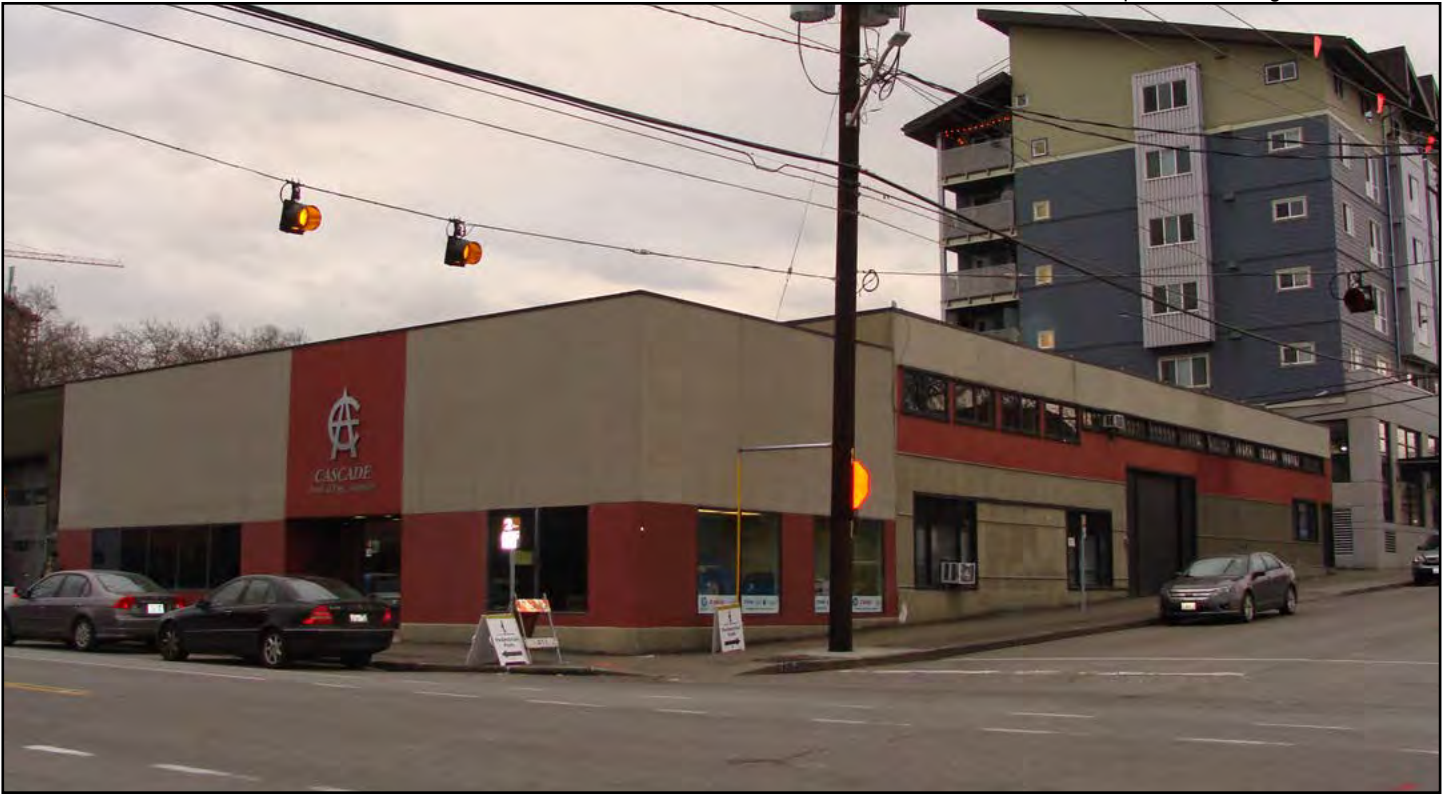
Figure 45 • Kuney Johnson General Contractor, altered (1945, now Cascade Architecture & Engineering)
