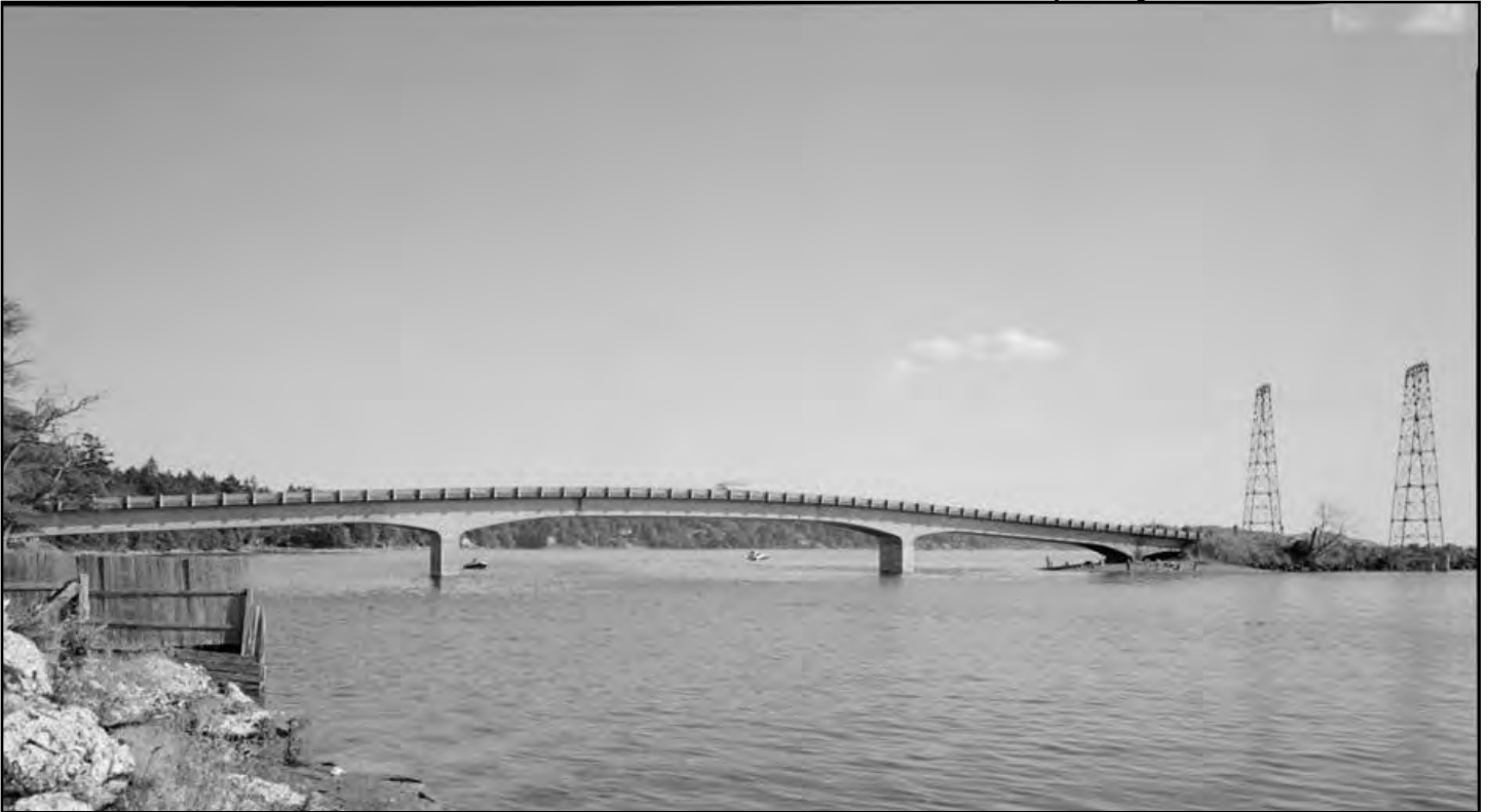
Figure 43 • Purdy Bridge (1936, George Runciman, engineer)
