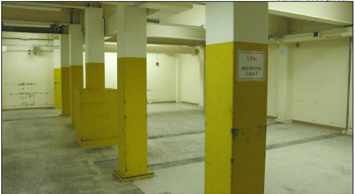
Figure 20 • Federal Reserve Bank, Seattle, interior of vault at basement
