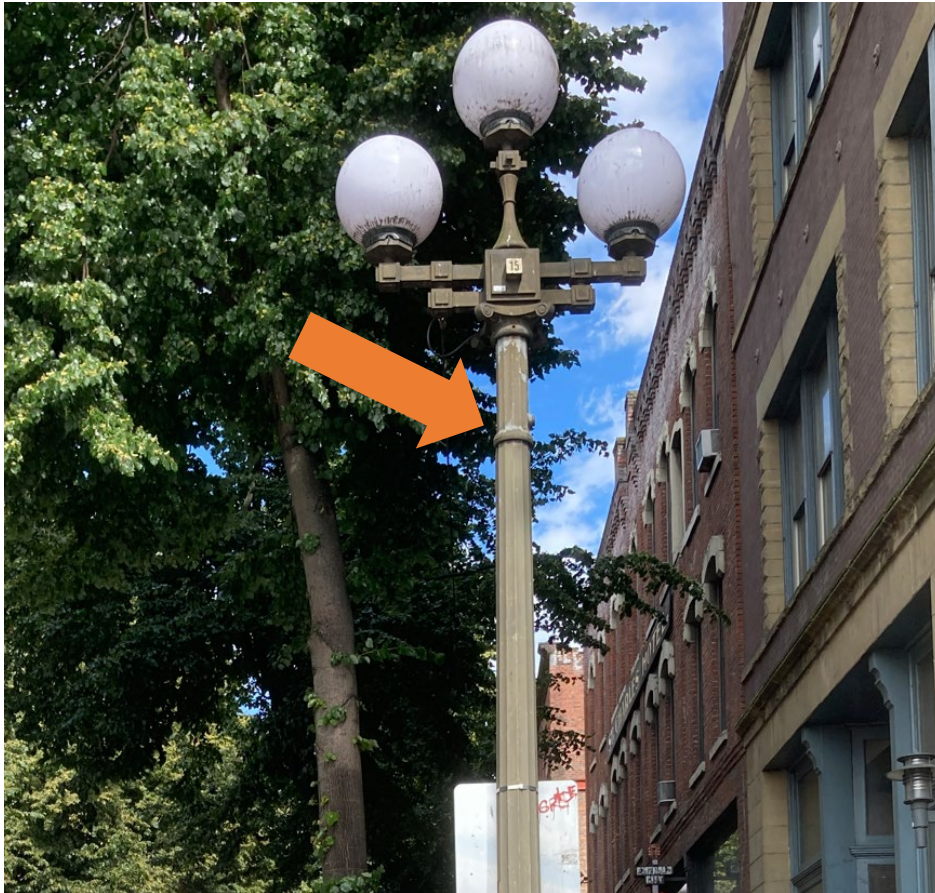
Figure 1. "Type D" pole with collar identified.
