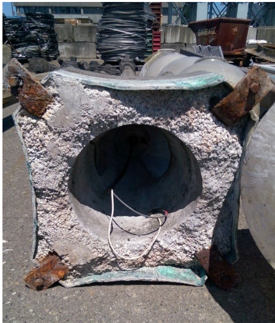
Figure 2. Example of Chief Seattle Base removed during construction
