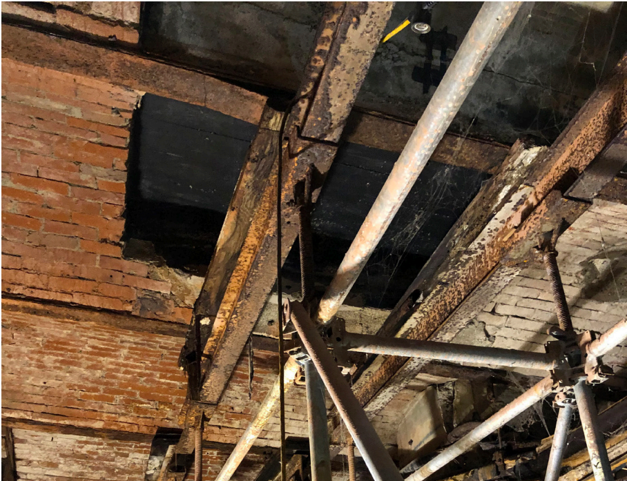
View of infilled skylights and temporary shoring supporting failing beams.
