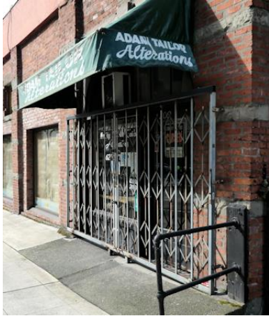
Figure xxx. Security bars and gates such as this detract from the area's pedestrian qualities and are prohibited.
