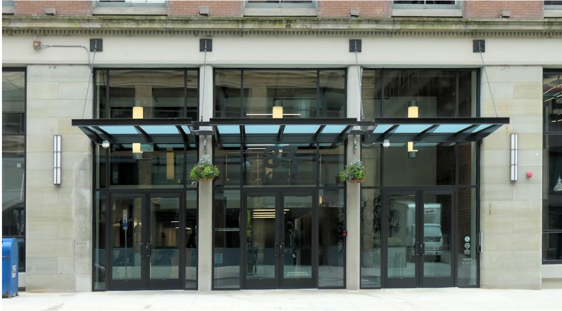
Figure xxx. Example of an appropriate storefront that has been replaced
