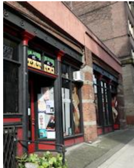
Figure xxx. Some buildings feature cast iron elements.
