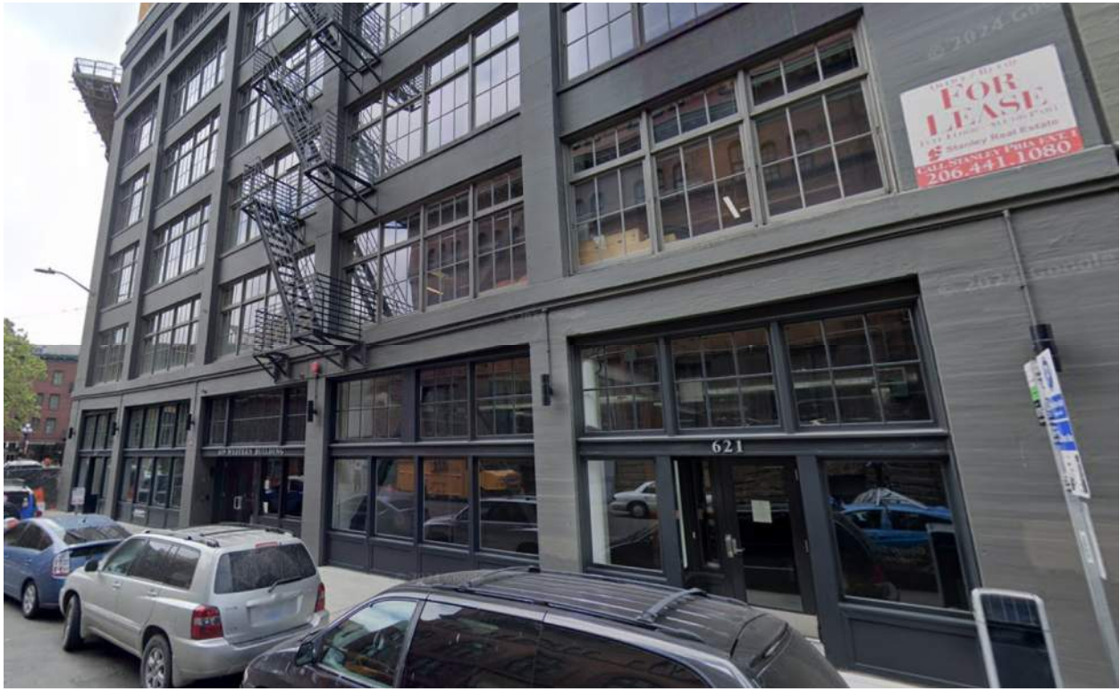
619 Western building from Western Avenue.
