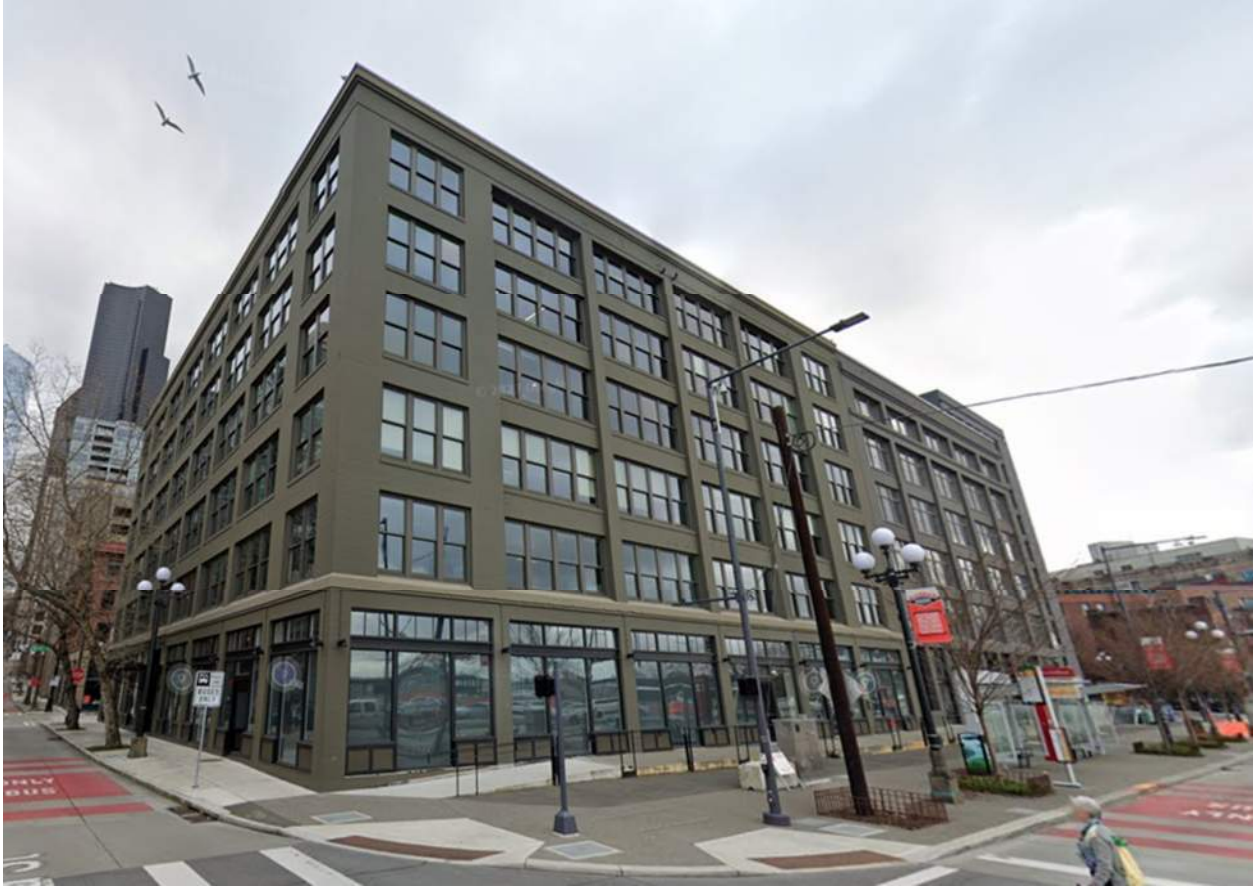
Looking east at the northwest corner of Polson Building.
