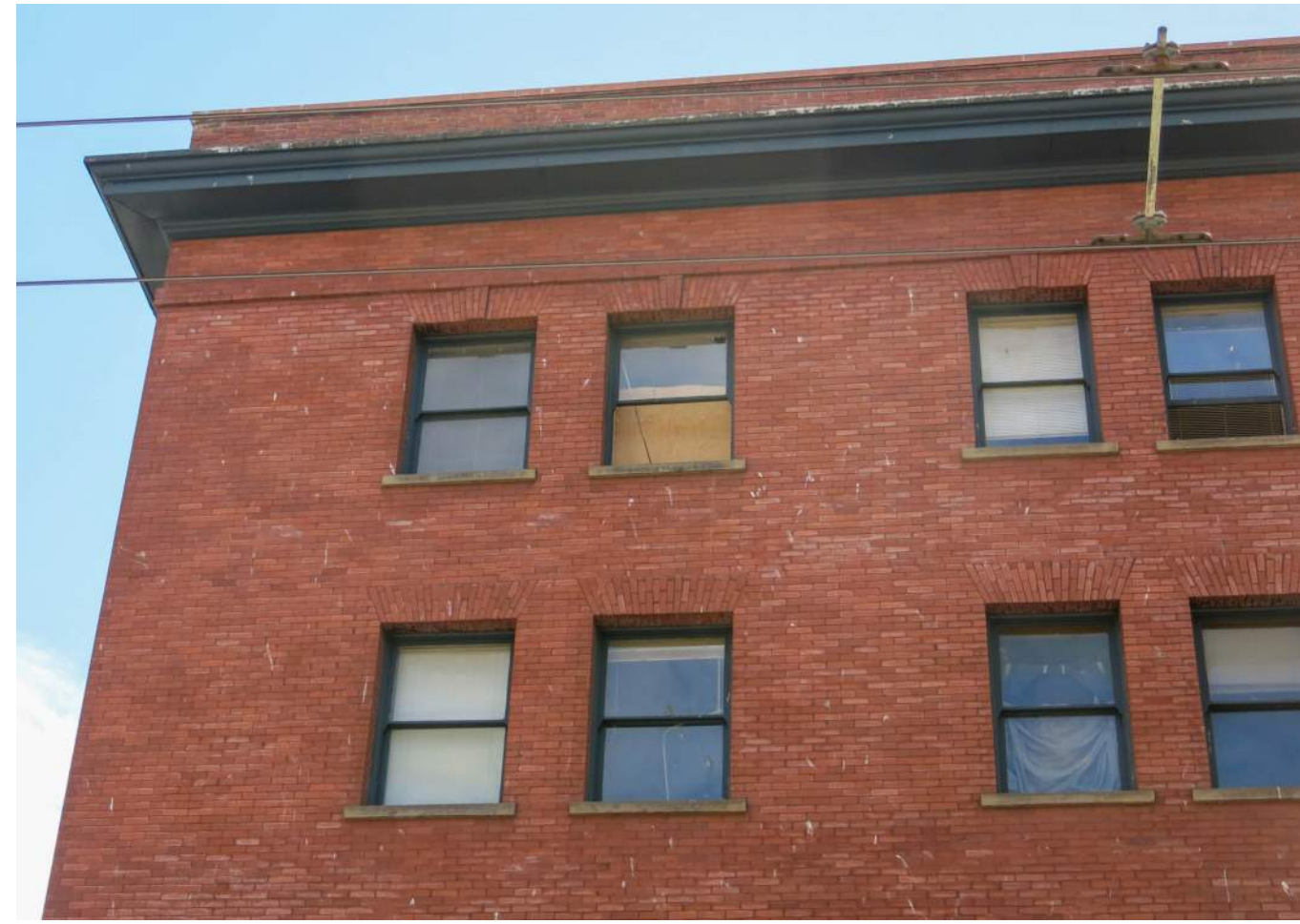
NORTH ELEVATION UPPER WINDOWS 2021
