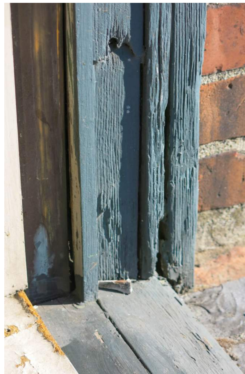
UNIT 411 WINDOW INTERIOR 2021
