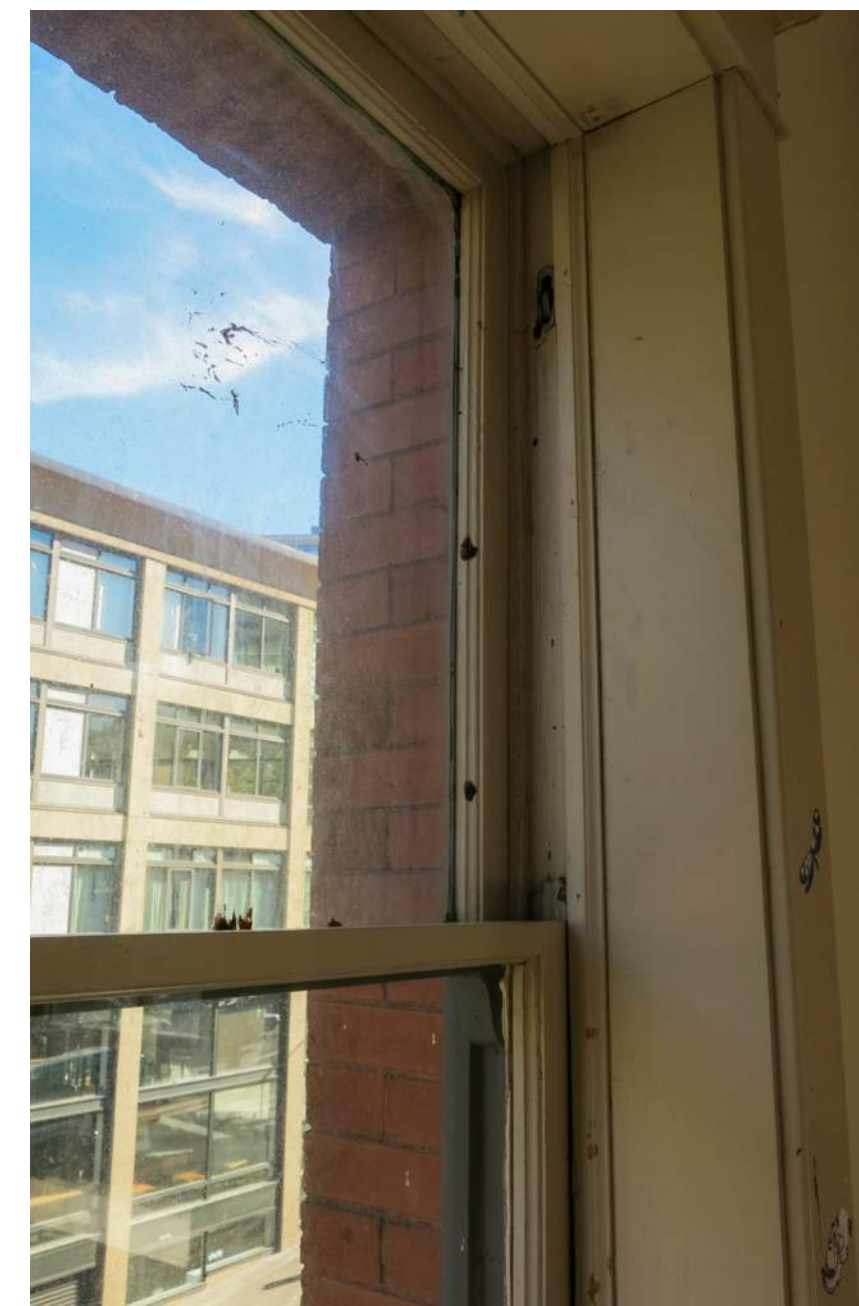
UNIT 411 WINDOW INTERIOR 2021
