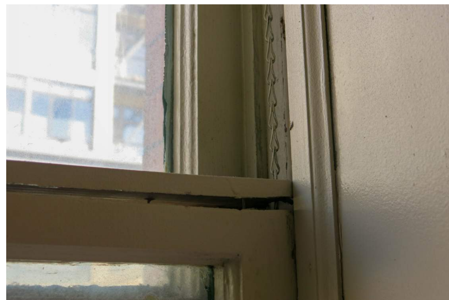
UNIT 215 WINDOW INTERIOR 2021
