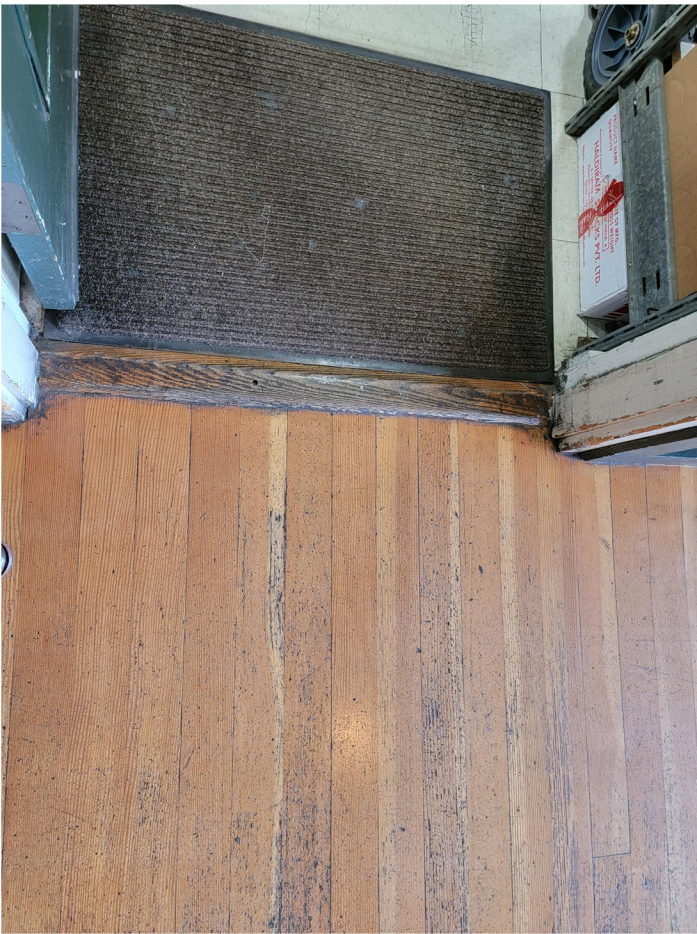
Floor Exposed wood and refinish to match wood floor @ hallway
