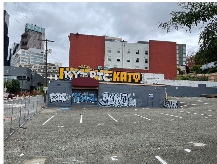
South elevation of existing building
