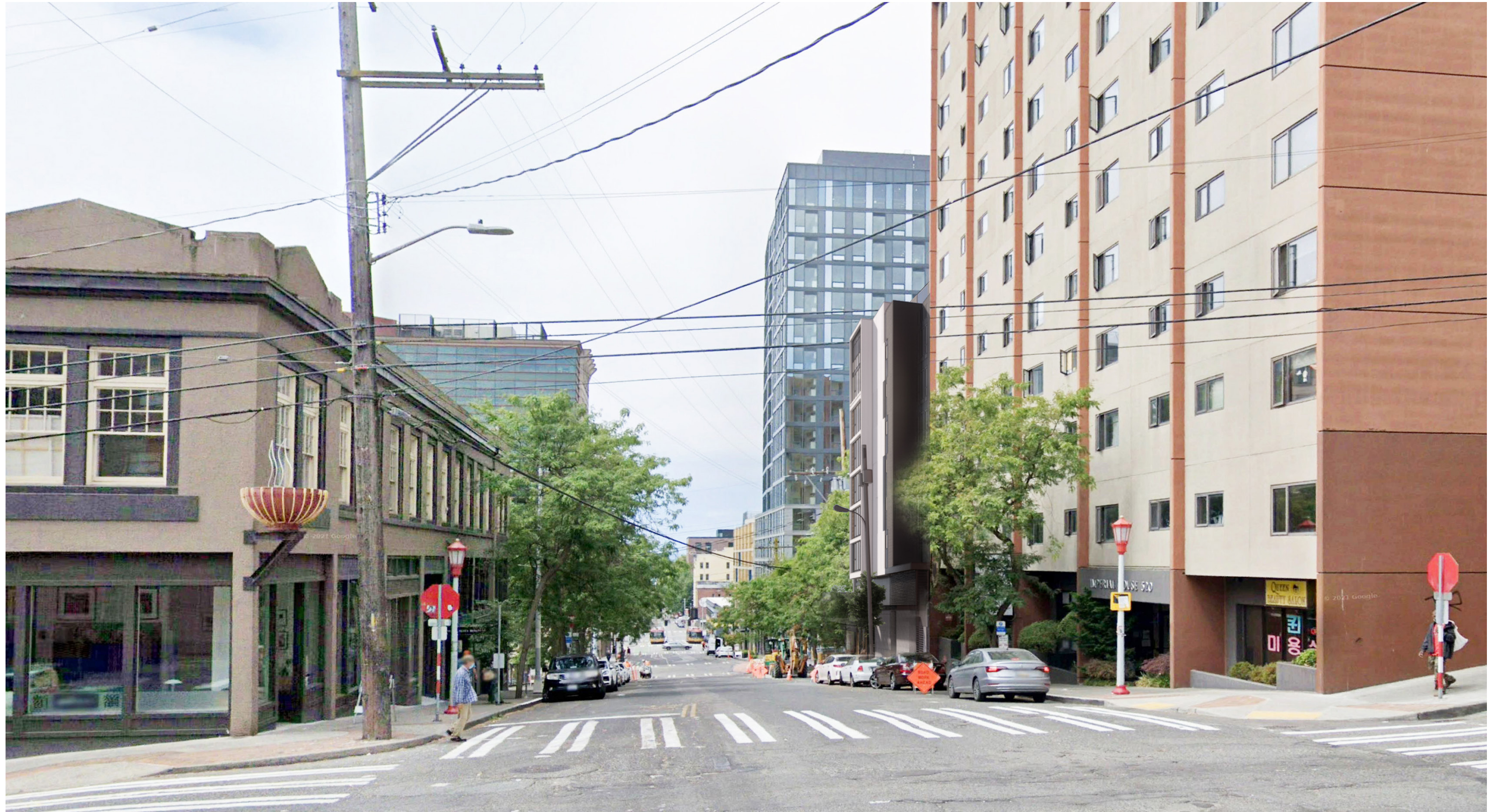
S MAIN ST. & 6TH AVE INTERSECTION FACADE
