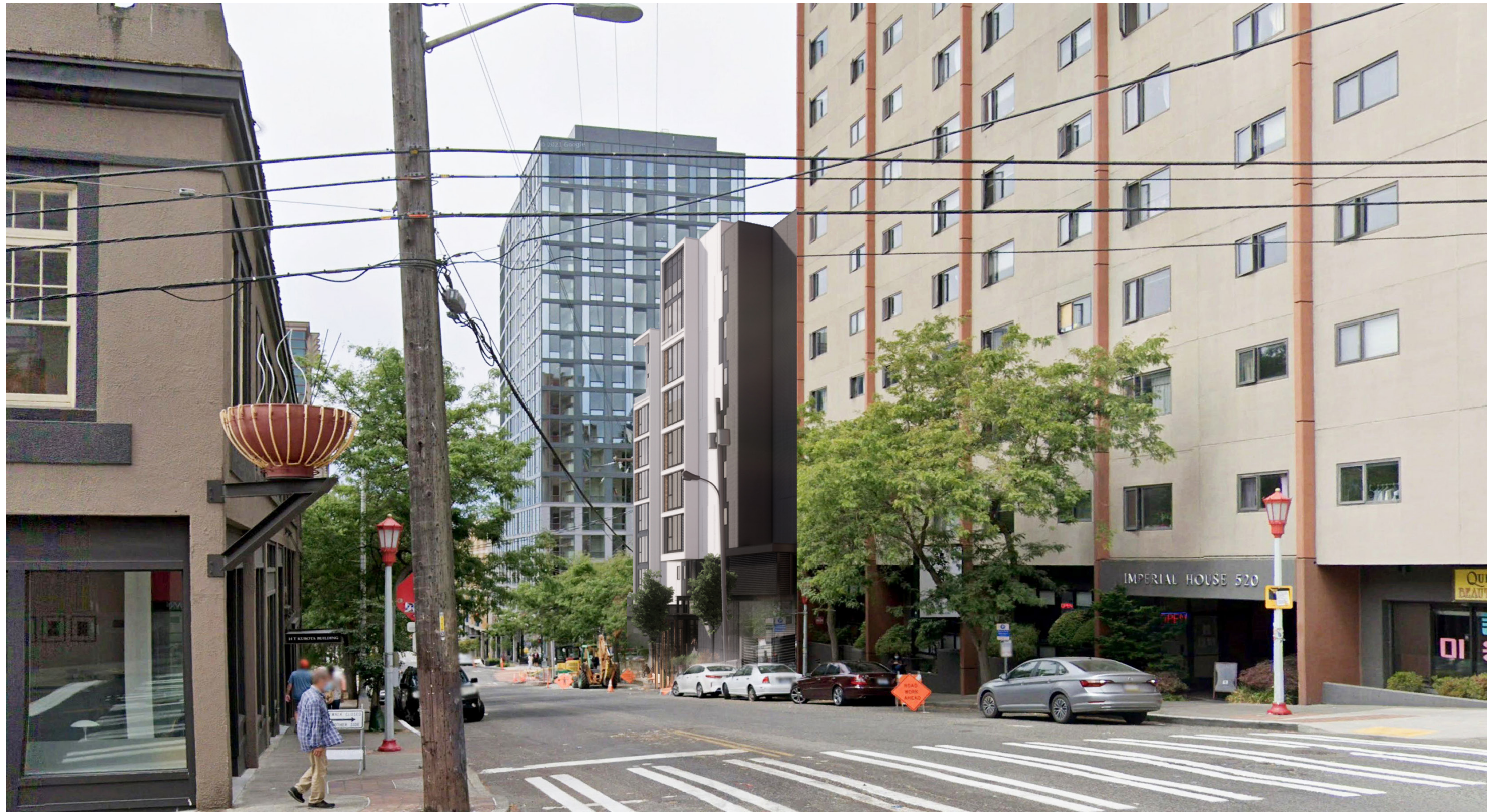
S MAIN ST. & 6TH AVE INTERSECTION FACADE
