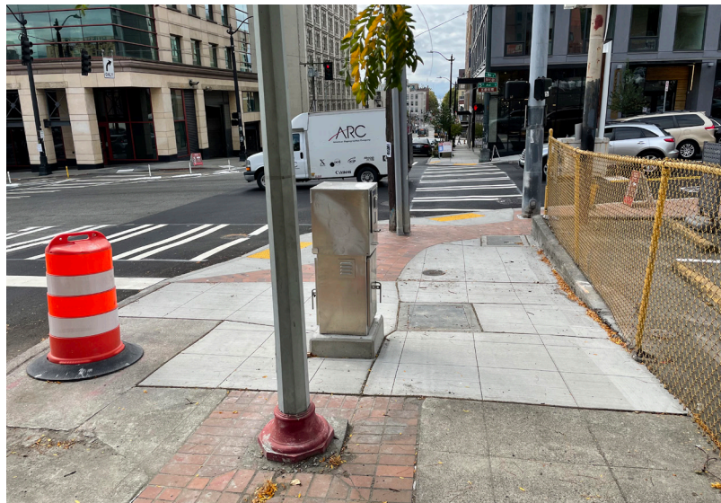
4. Street Lamp and electrical transfer box
