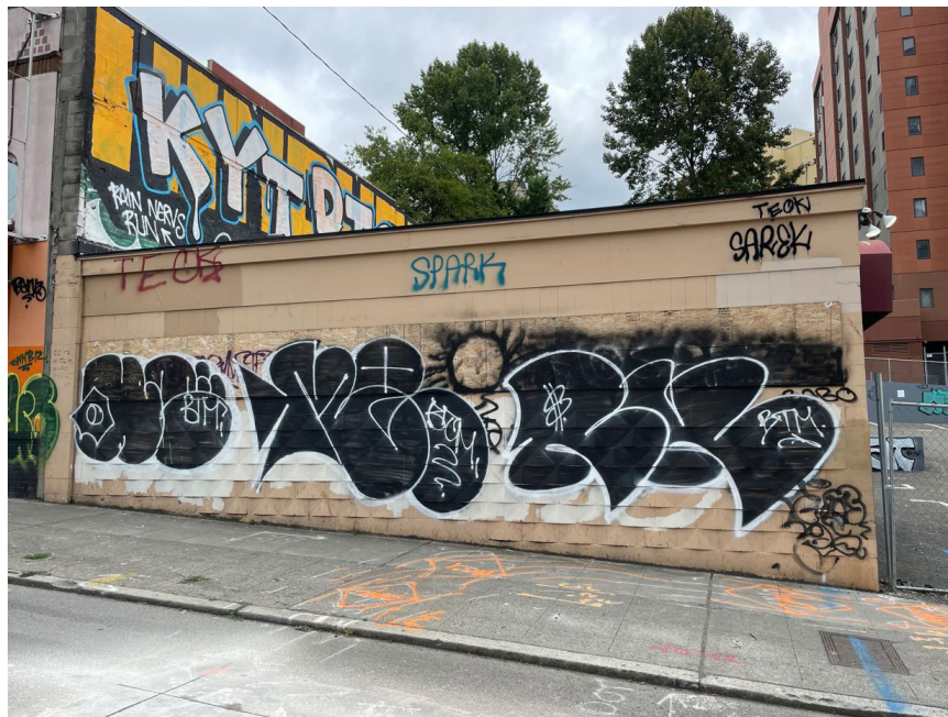
West elevation of existing building
