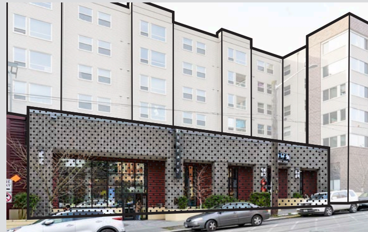
Podium with entrances at ground level and setback mass above to create a terrace (pictured: S Lane St and 8th Ave S, International District/Chinatown Branch - The Seattle Public Library)
