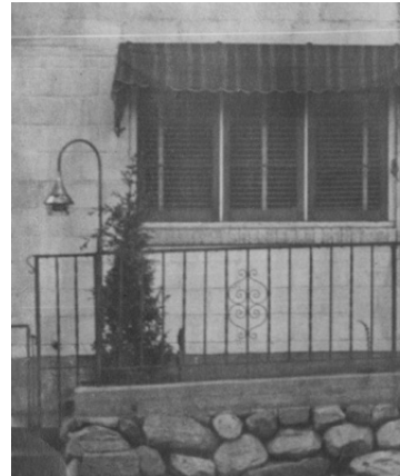
Wrought iron - repaired or reconstructed to match historic images
