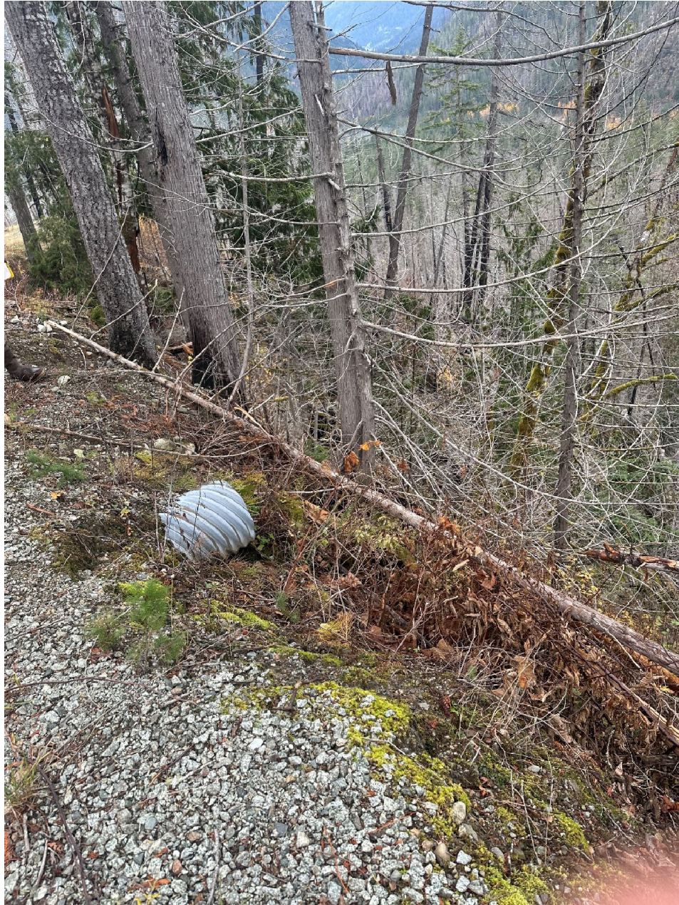
Photo 1. Culvert 11 outlet. Stream 1 flows through Culvert 11 and immediately discharges over a 6-foot drop onto boulders. From there, it has a steep slope (15 to 20 percent) for approximately 20 feet, and then flows over a near vertical drop to Newhalem Creek.
