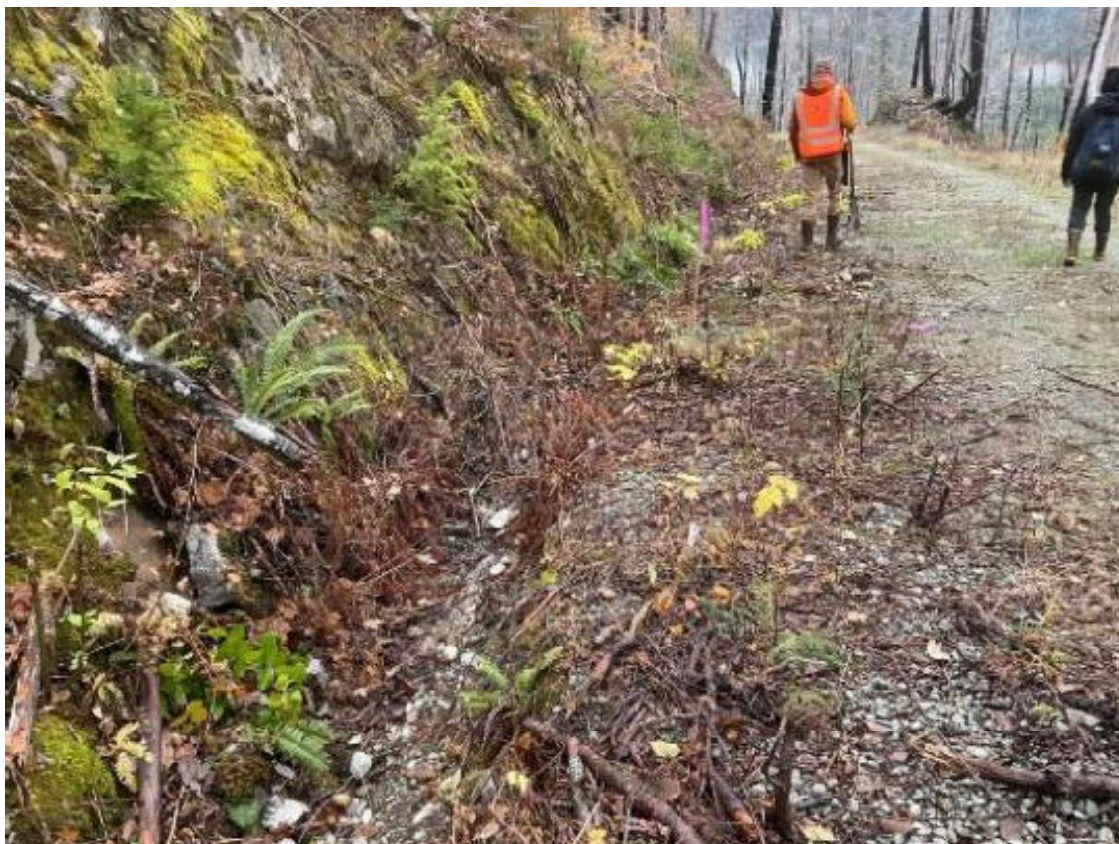
Photo 7: Ditch 2, located approximately 10 feet west of Culvert 12. Ditch 2 is an excavated roadside feature that conveys stormwater northwest along the dam access road. The bed and bank of the ditch are comprised of quarry spall and gravel, with scattered upland vegetation.
