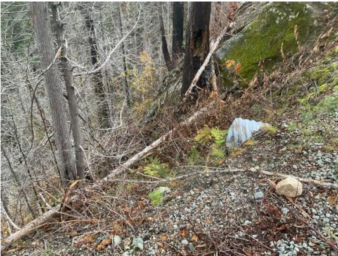
Photo 6: Culvert 12 outlet. Expressed groundwater and stormwater runoff from Ditch 1 flows through Culvert 12 and is discharged to the top of a steep slope/cliff. Immediately after the cliff and outside of the study area, the conveyed flow goes subsurface and lacks a downstream connection to Newhalem Creek.
