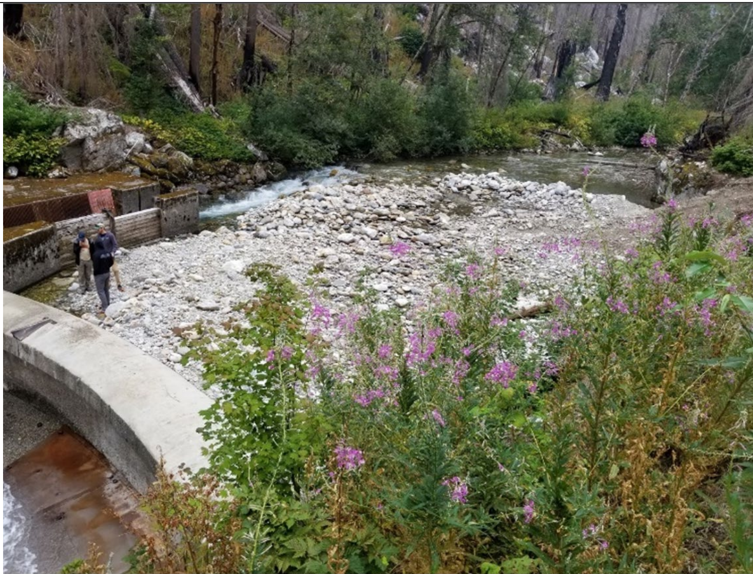
Newhalem Dam, August, showing low flow conditions, looking upstream. Creek flows along right bank into sluiceway; left bank “in the dry.”
