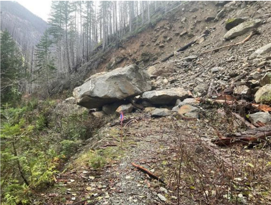
Photo 1: Landslide on dam access road as of November 2023. Photo taken facing SW from dam access road.
