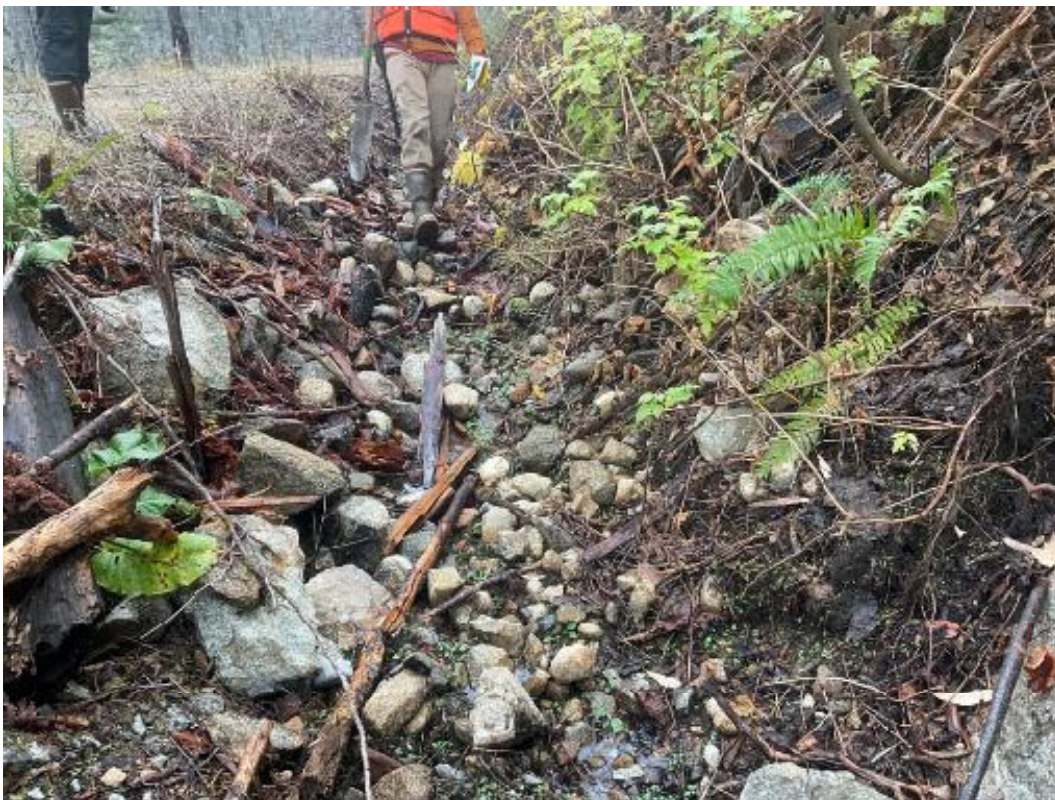
Photo 4: Ditch 1, comprised of quarry spall and scattered upland vegetation. Photo taken facing SE.
