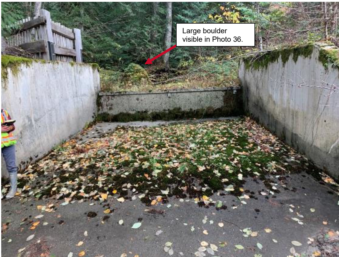
Photo 37: Tailrace barrier. Photo taken facing upstream (south) into the tailrace from the left bank of the Skagit River.
