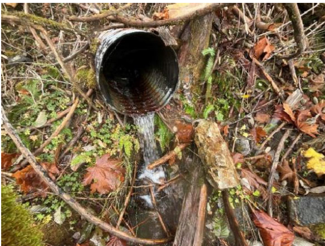
Photo 14: Culvert 11 outlet, located on the north side of the dam access road. Water conveyed through the culvert discharges onto large boulders and drops approximately 6 feet below the culvert.
