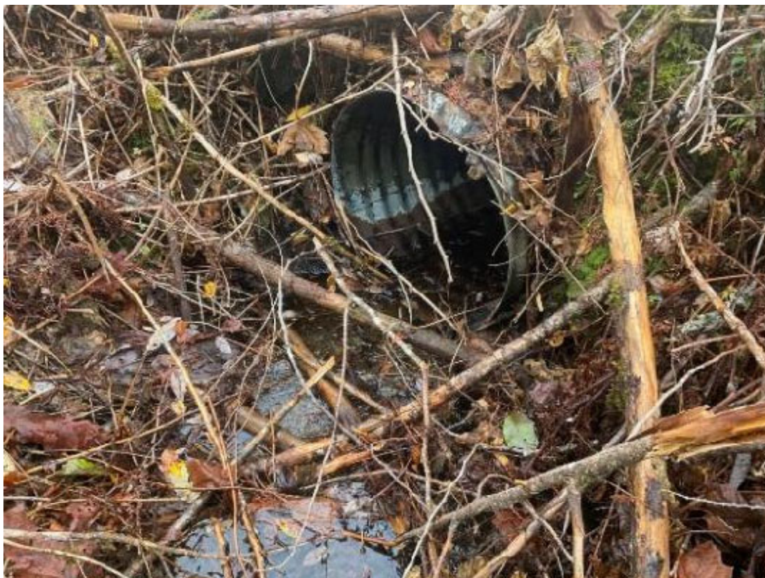
Photo 13: Culvert 11 inlet, located on the boundary of Wetland 1. Culvert 11 conveys Stream 1 under the dam access road.
