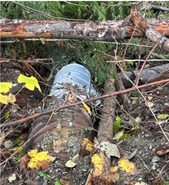
Photo 2: Culvert 13 outlet. Culvert 13 is a perched culvert located underneath the dam access road just downslope of the landslide area. The inlet to Culvert 13 appears to be buried and was not visible during the site investigation in November 2023.
