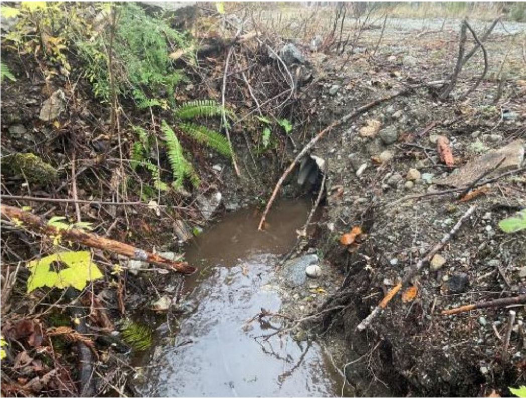
Photo 5: Culvert 12 inlet, containing expressed groundwater and hillside seeps conveyed in Ditch 1.
