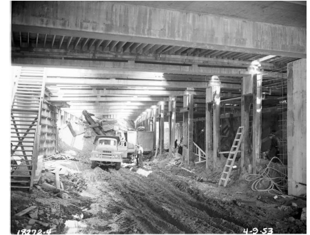
Battery Street Tunnel under construction, April 9, 1953.
