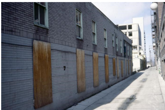
Stewart House and Post Alley [Pike Place Market rehabilitation], circa 1977 Item 192053 , (Series 1629-01), SMA.
