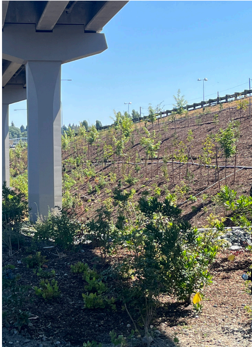
Restoration near Lightrail bridge at NE Northgate Way / 1st Ave NE
