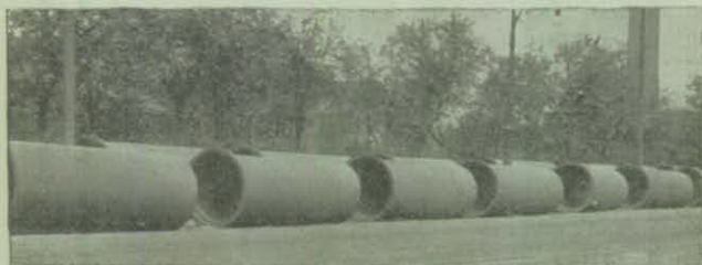
Pipe Strung Along Street Ready for Laying
