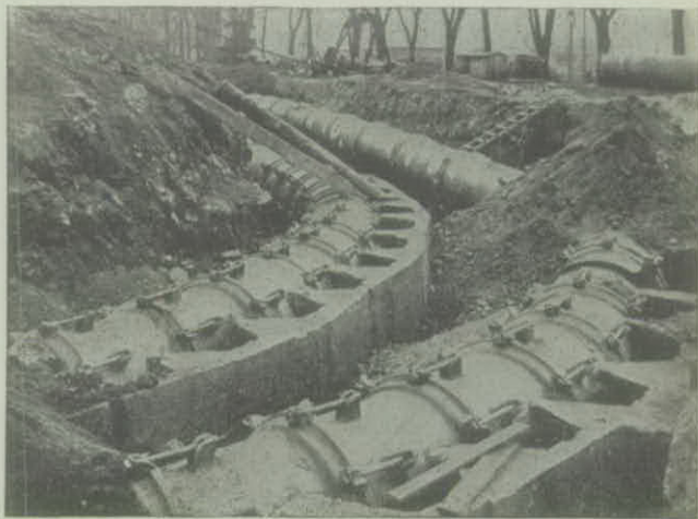
Lugged Bends Reinforced with Masonry Piers
