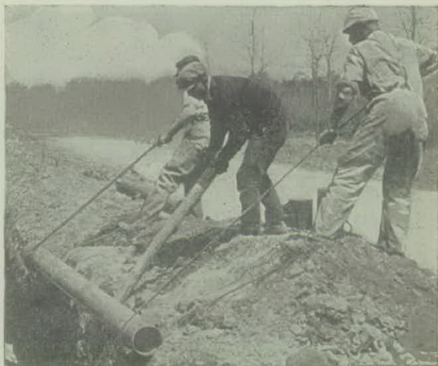
Lowering Small Pipe Into Trench by Hand
