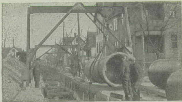
Special Gantry Crane for Laying Large Pipe
