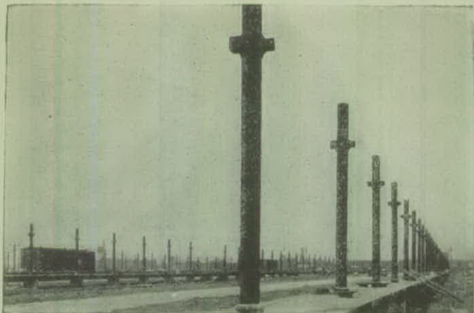
Cast Iron Pipe Columns in Warehouse Construction
