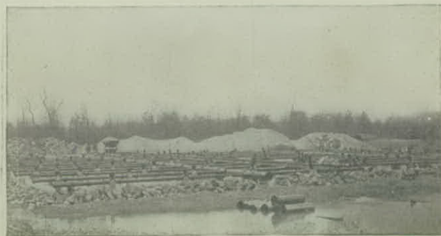
In a Sewage Disposal Plant
