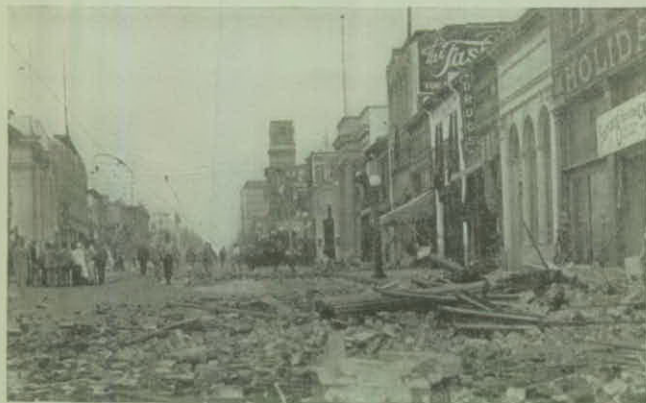
Effect of Santa Barbara Earthquake on Surface Structures
