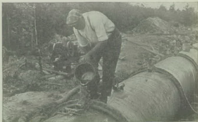
Pouring a Bell and Spigot Joint with Leadite
