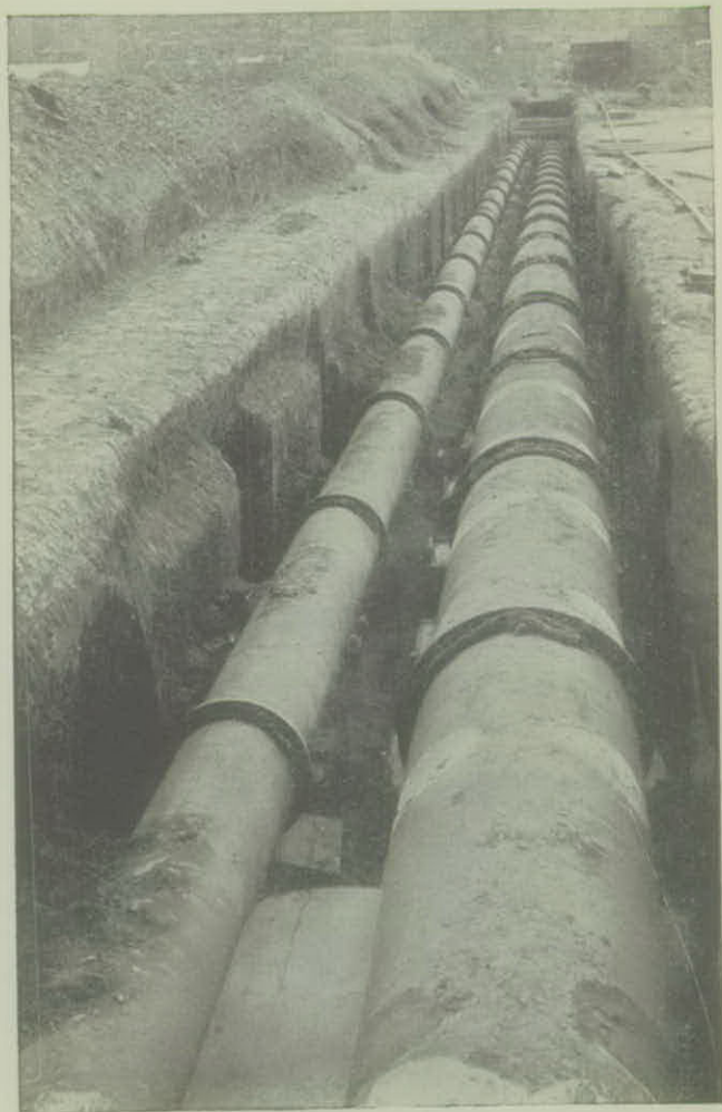
A 36-inch and a 20-inch Bell and Spigot Gas Line in the Same Trench
