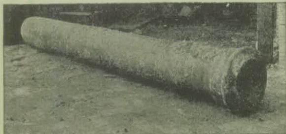
Earliest Cast Iron Gas Pipe after 80 Years of Service in Baltimore
