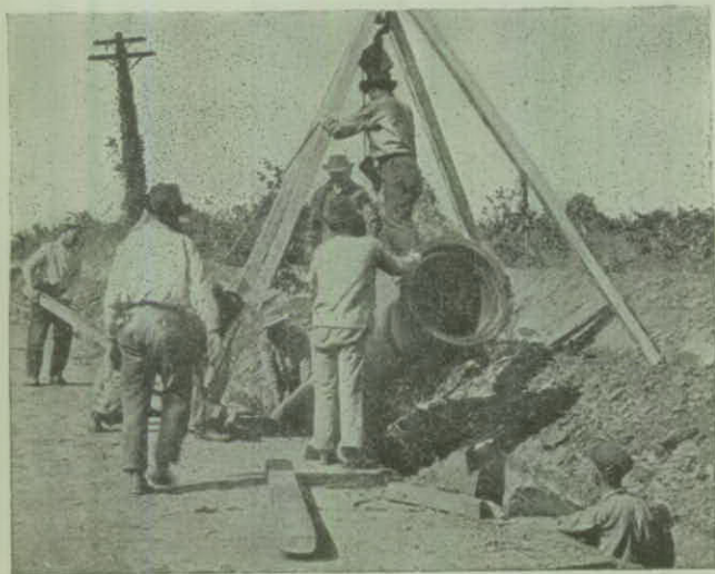
Tripod for Lowering Large Pipe into Trench
