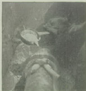
Pouring a Lead Joint, Showing Runner in Place
