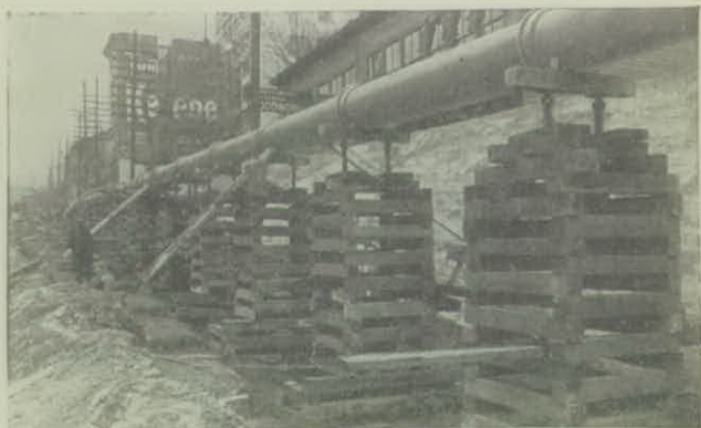
Raising a Bell and Spigot Water Line Under 120 Pounds Pressure
