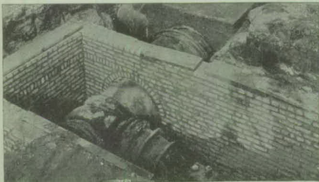
Valve Vault Under Construction
