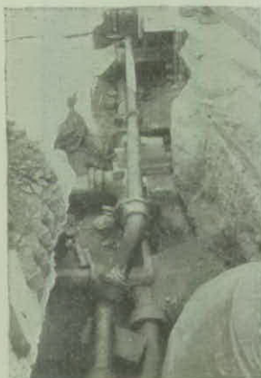
An Intricate Installation of Gas and Water Lines
