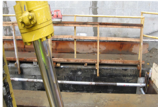
Figure 3-13 Trench Side View
