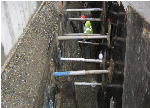
Figure 3-12 Excavation Next to a Building
