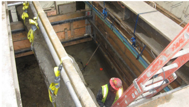
Figure 3-9 Beam and Strap Utility Support
