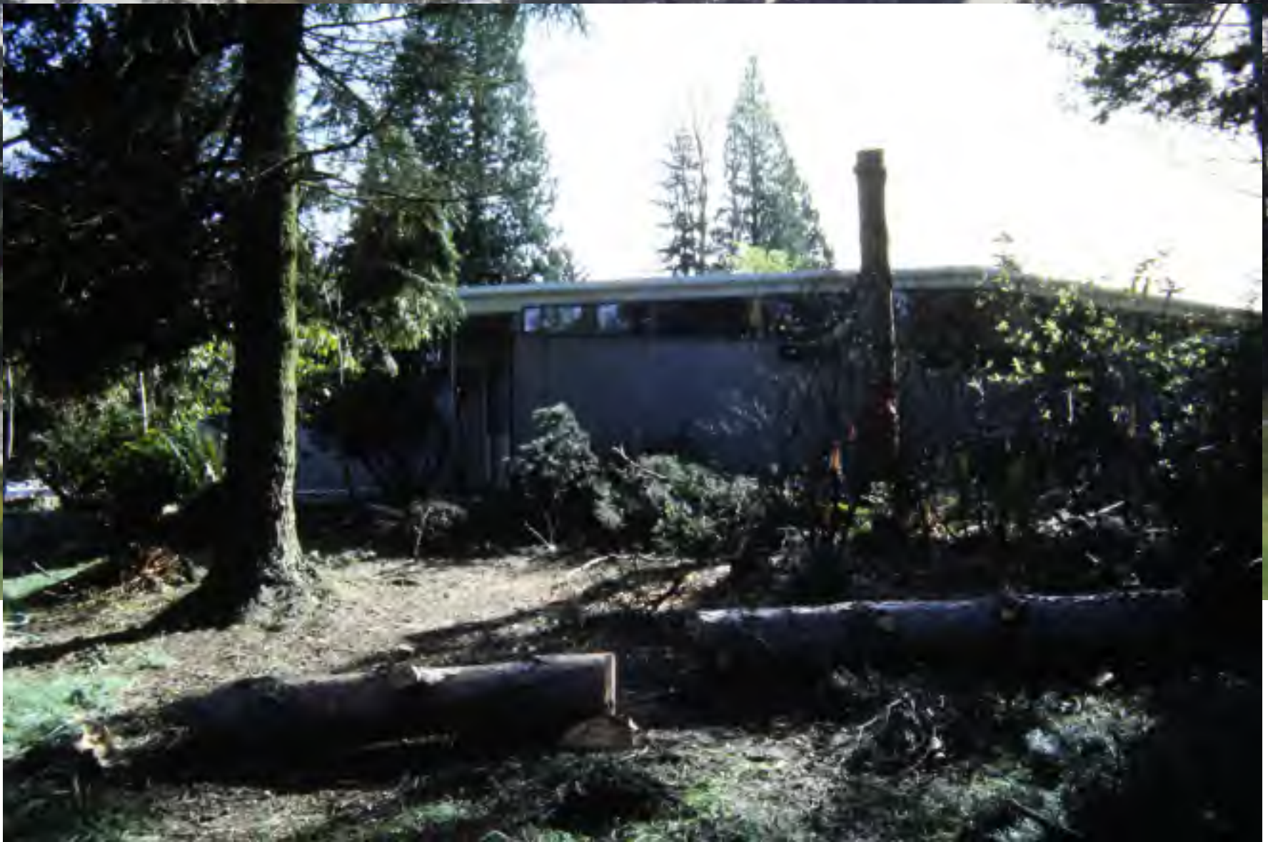
North side “back” of the Visitor’s Center
