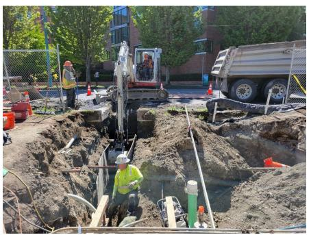
Figure 3-2. Force Main Replacement at Wastewater Pump Station 62
