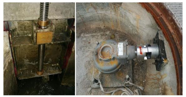
Figure 4-1. New Basin 99 Sluice Gate (Left) and Actuator Motor (Right)
