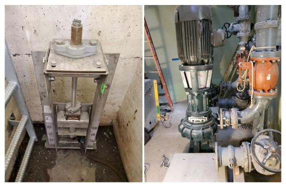
Figure 4-4. Installation of Basin 138 Slide Gate (Left) and New Higher Capacity Pumps (Right)
