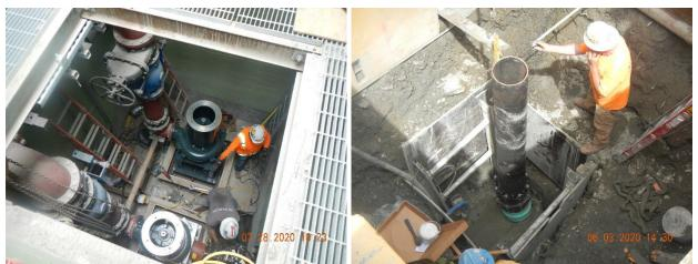
Figure 4-2. New Basin 60 Pumps Being Installed (Left) and New Basin 60 Connection to King County Trunk Sewer (Right)
