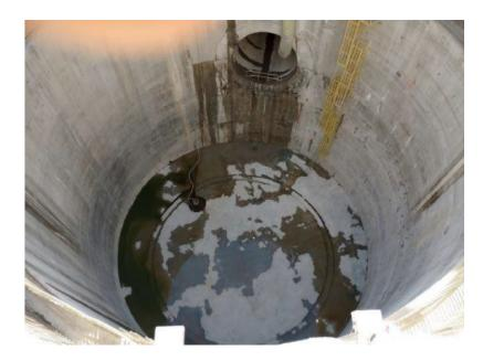
Figure 4-6. 8 ft. Drop Shaft in Ballard, Ready for Pump Station Construction
