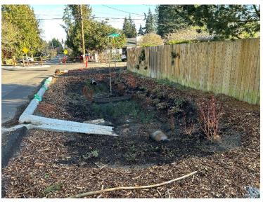
Figure 4-12. Looking East from 24th Ave SW and SW Kenyon St – The New Bioretention Facility, Walkway, and Bridge
