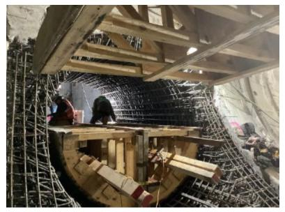
Figure 4-5. Construction of a Connector Tunnel Between Storage Tunnel and Drop Shaft
