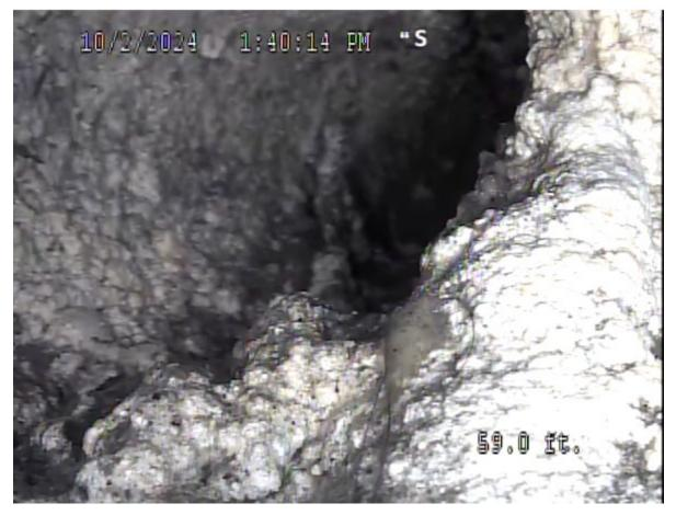
Figure 3-1. 2024 Mainline Image Demonstrating Visible FOG Accumulations Resulting in SSO Near the University of Washington
