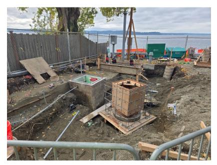
Figure 3-6. Site Work in Progress at Wastewater Pump Station 71
