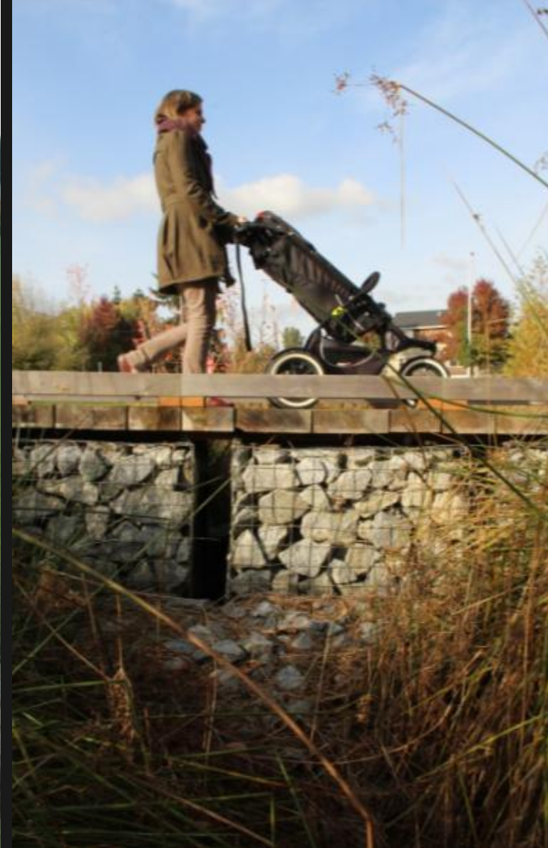
gabion bridge crossing
