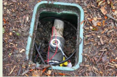
Flow Sensor in Ground
