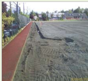
Making Drainage Repairs
