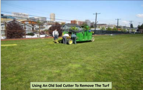
Using An Old Sod Cutter To Remove The Turf
