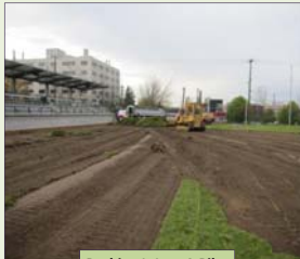
Pushing It Into A Pile
