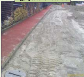
Digging Out 8" Of Root Zone
